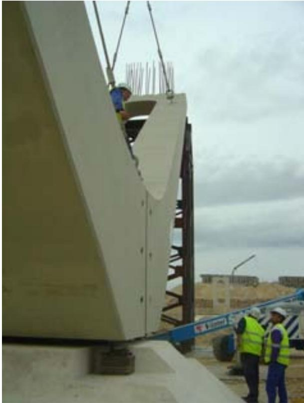
*Fig 8 Pila colocada.*
