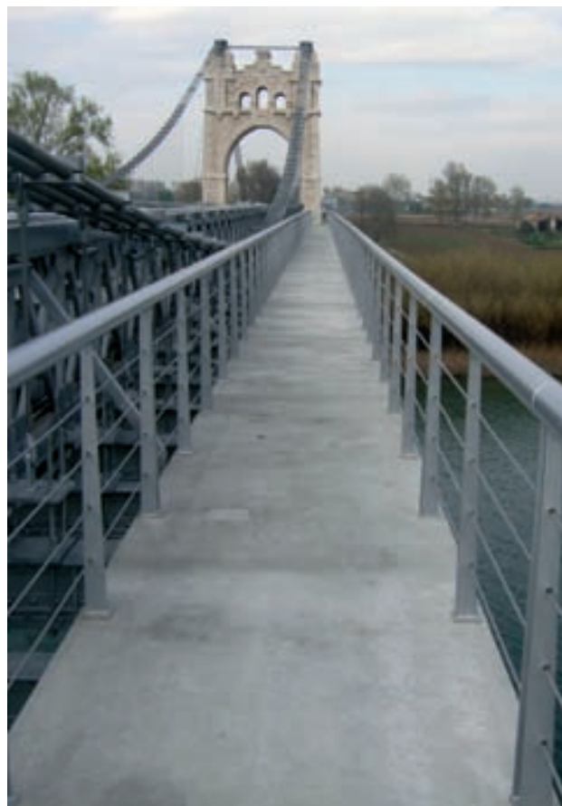
Figura 40. Nueva acera terminada. Figure 40. Finished walkway.
