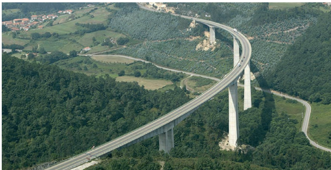
Figura 2. Viaducto original Figure 2. Existing bridge
