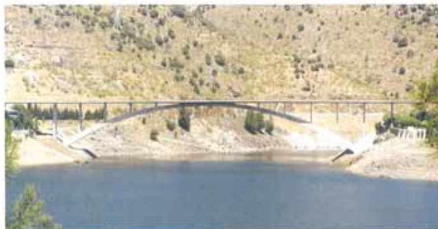
Foto 1. Vista general del arco. Picture 1. General view of the bridge.
