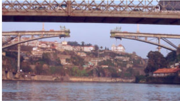
**Fig. 6: Unión arco-dintel**
