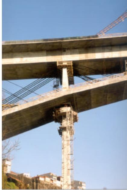
**Fig. 8: Pila provisional**
