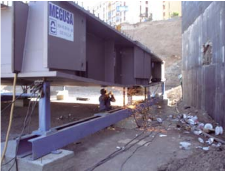
Figura 16. Diafragma de estribo 1. Figure 16. Diaphragm of abutment 1.
