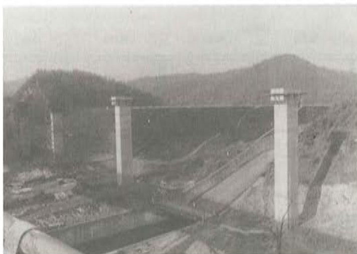
Fig. 4. KEUM GOK CHUN BRIDGE Pilas centrales
