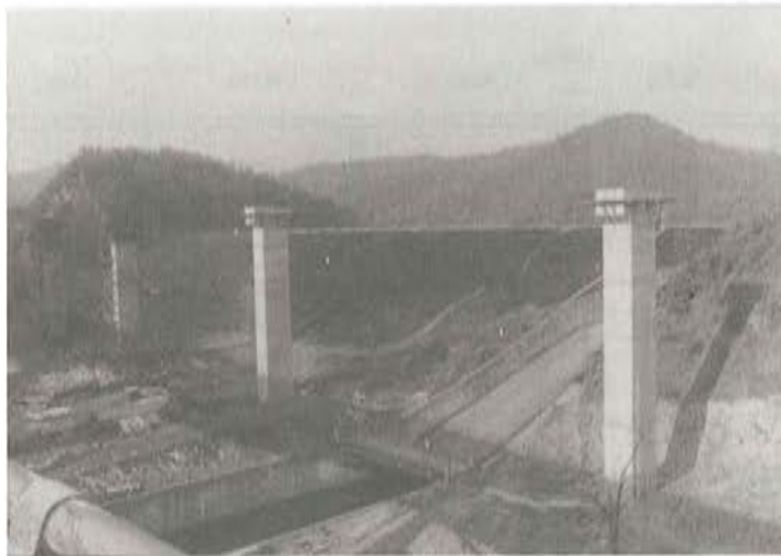
Fig. 4. KEUM GOK CHUN BRIDGE Pilas centrales
