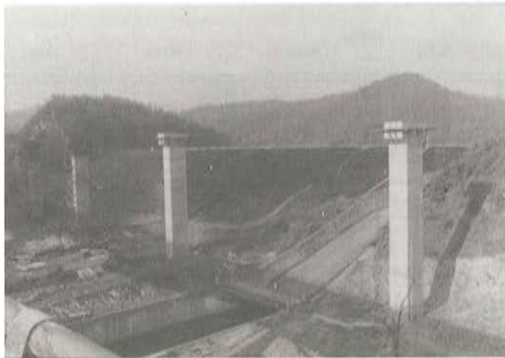
Fig. 4. KEUM GOK CHUN BRIDGE Pilas centrales
