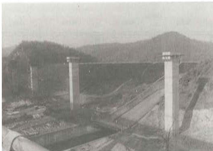
Fig. 4. KEUM GOK CHUN BRIDGE Pilas centrales
