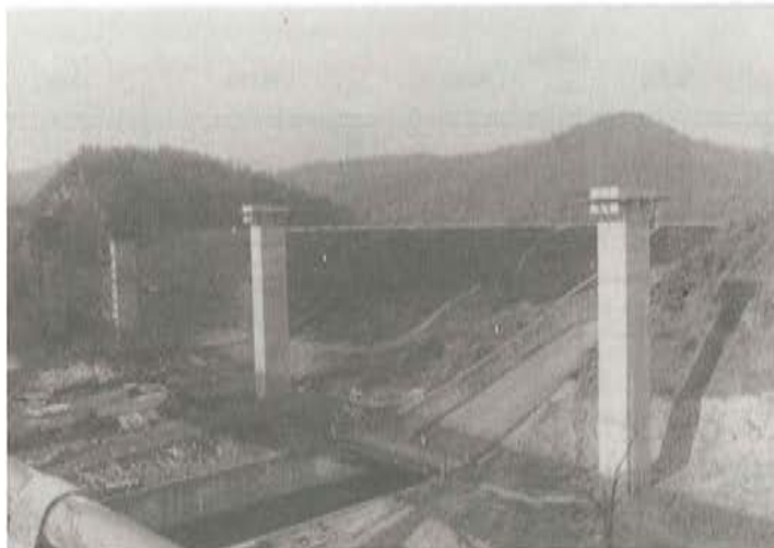
Fig. 4. KEUM GOK CHUN BRIDGE Pilas centrales
