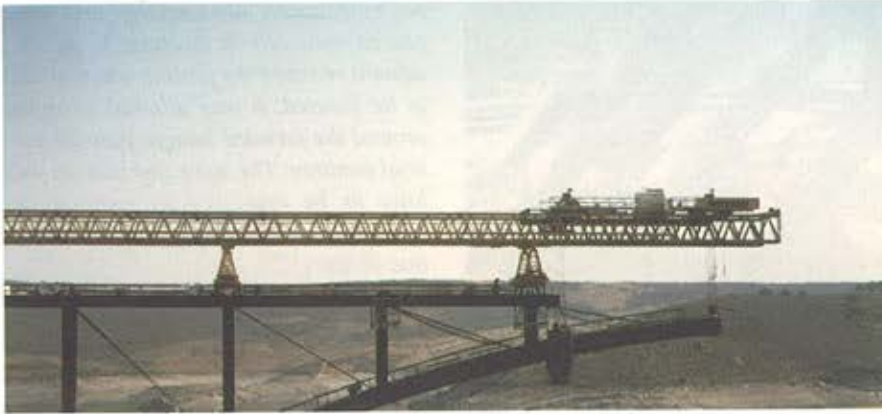
Figura 32. Voladizo del semiarco de la margen derecha. Figure 32. Half-arch cantilevering on right-hand bank
