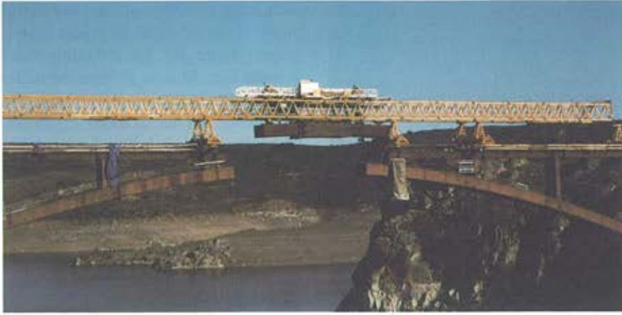
Figura 34. Lanzamiento del tramo de clave. Figure 34. Carrying out the key segment.
