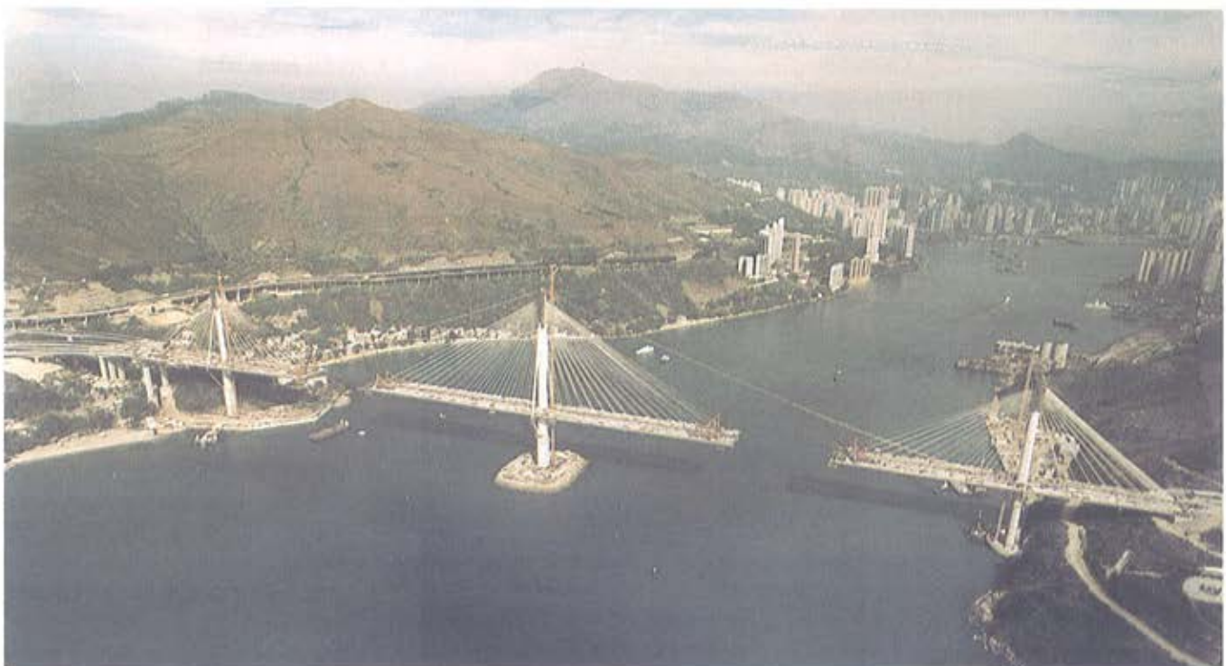
Figura 22. Montaje del tablero. Vista general. Figure 22. Deck erection. General view.
