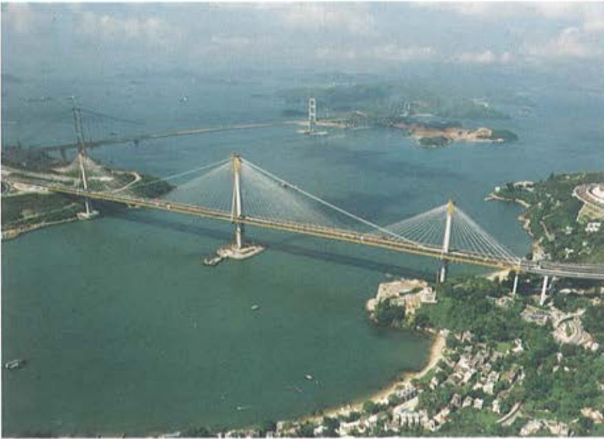
Figura 1. Vista general del puente. Figure 1. General view of the bridge
