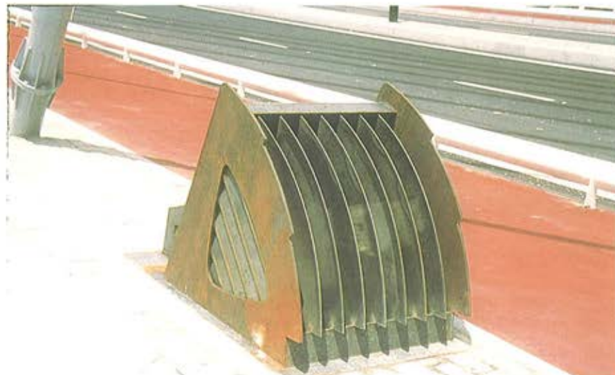
Figura 17. Concha de acero corten para alojar focos de iluminación. Figure 17. Shell of weathered steel provided for sheltering the lamps of artistic lightning.
