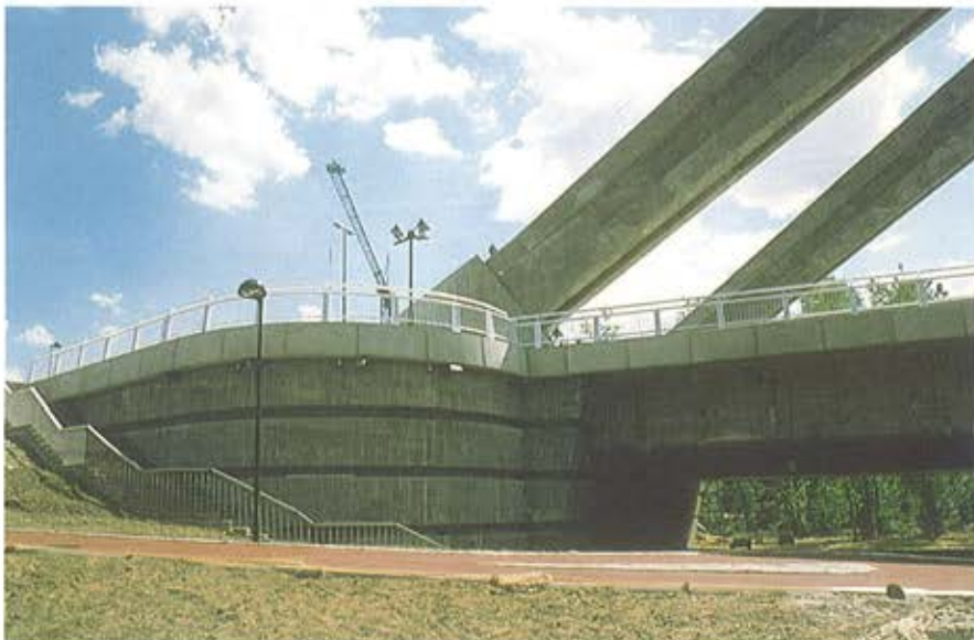
Figura 15. Vista del contrapeso final con los arranques de velas en el puente acabado. Figure 15. View of the final block of counterweight with the beginning of the inclined sails.
