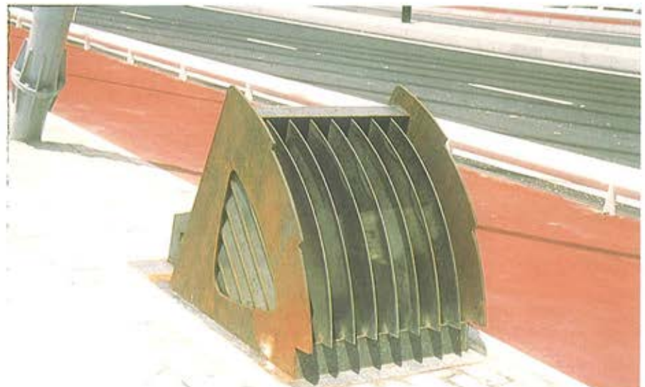
Figura 17. Concha de acero corten para alojar focos de iluminación. Figure 17. Shell of weathered steel provided for sheltering the lamps of artistic lighting.
