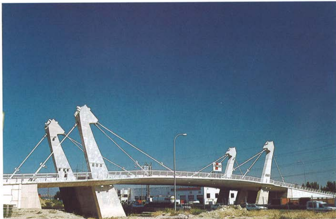
Figura 19. Vista general del puente terminado. Figure 19. General view of the bridge finished.
