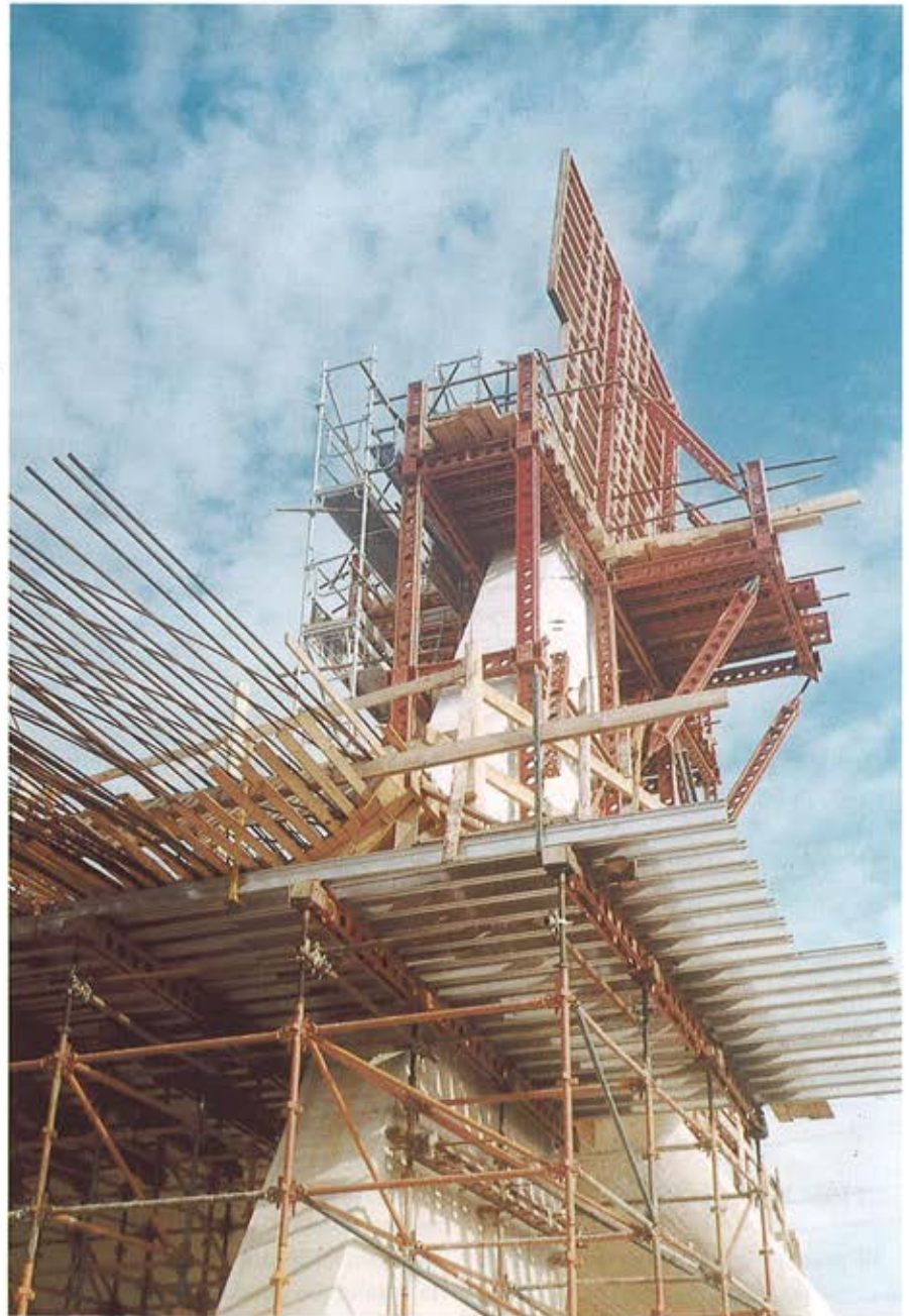
Figura 17. Vano lateral descimbrado Figure 17. Lateral span with falsework already dismantled.
