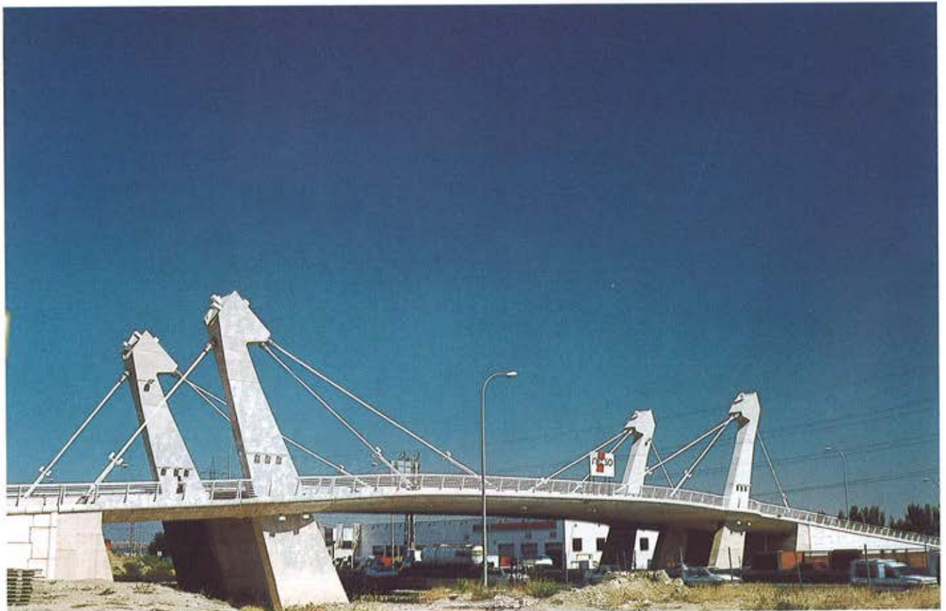
Figura 19. Vista general del puente terminado. Figure 19. General view of the bridge finished.
