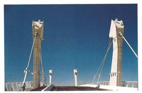
Figura 5. División del tablero en acera, carril-bici y calzada. Figure 5. Deck sections: Sidewalk, bicycle lane and rood way.
