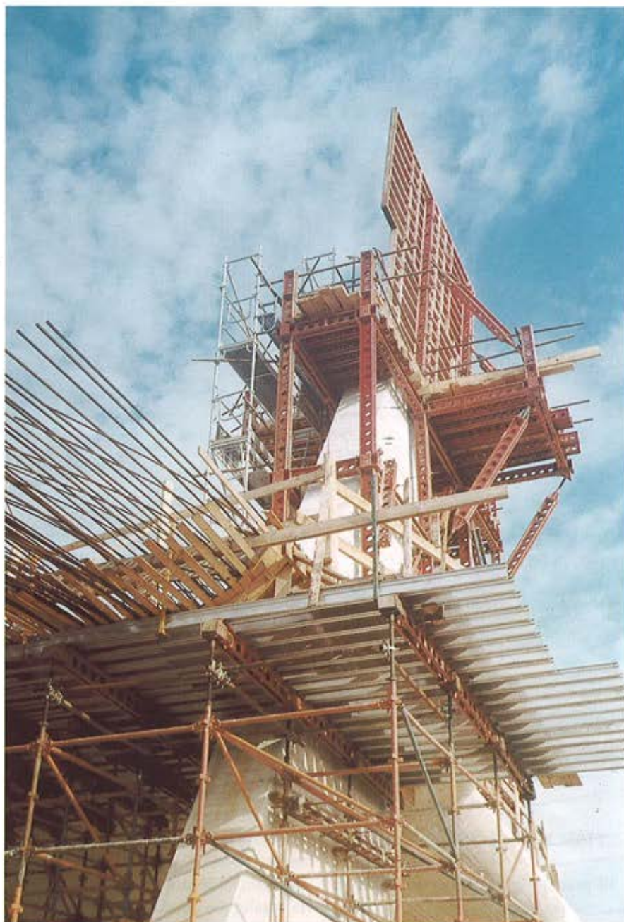
Figura 17. Vano lateral descimbrado Figure 17. Lateral span with falsework already dismantled.
