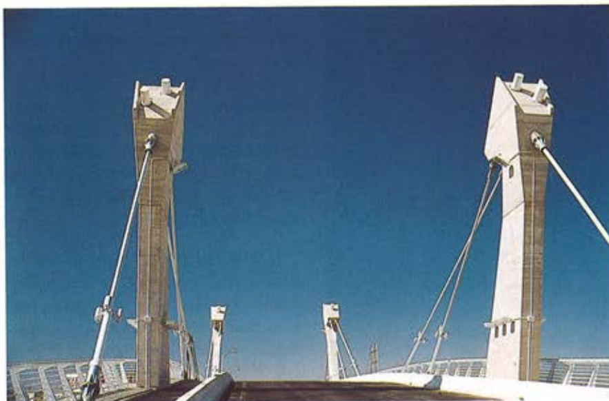
Figura 5. División del tablero en acera, carril-bici y calzada. Figure 5. Deck sections: Sidewalk, bicycle lane and roadway.
