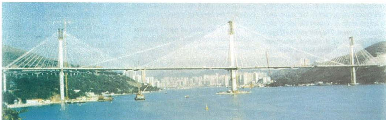
Figura 38. Vista del puente de Ting Kau (Hong Kong) Figure 38. View of Ting Kau bridge (Hong Kong).
