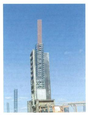
Figura 3. Detalle cabeza pilar mixto. Figure 3. Detail of head of composite columm.
