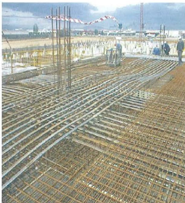
Figura 17. Vista general pretensado de planta primera. Figure 17. General view of prestressed slab.
