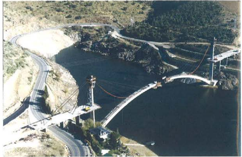
Foto 3. Vistas del arco durante procedimiento constructivo. Picture 3 Views of the arch during the construction procedure.
