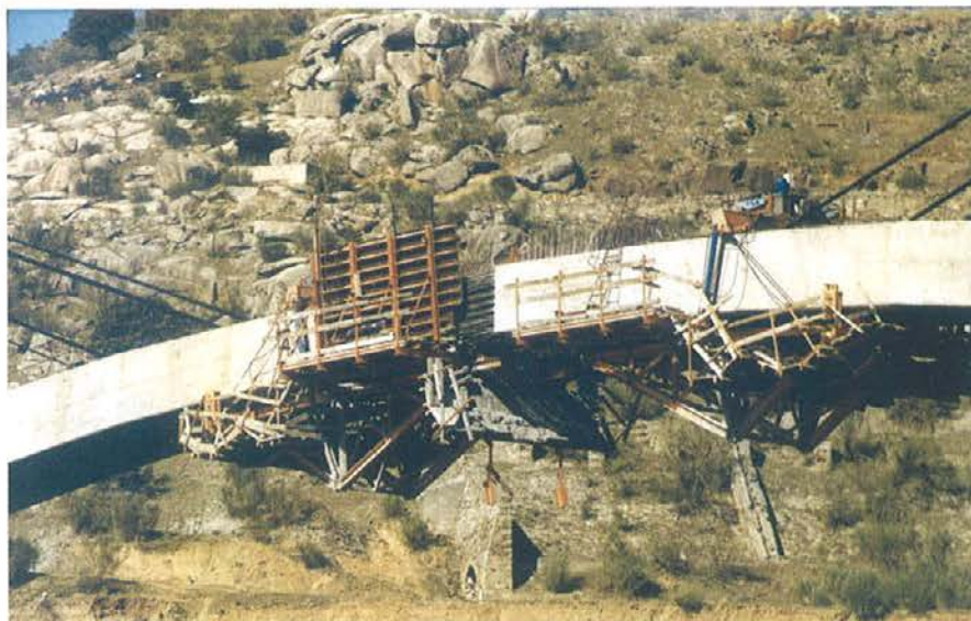
Foto 4. Vistas de los carros de avance. Picture 4. Views of travelling formwork.
