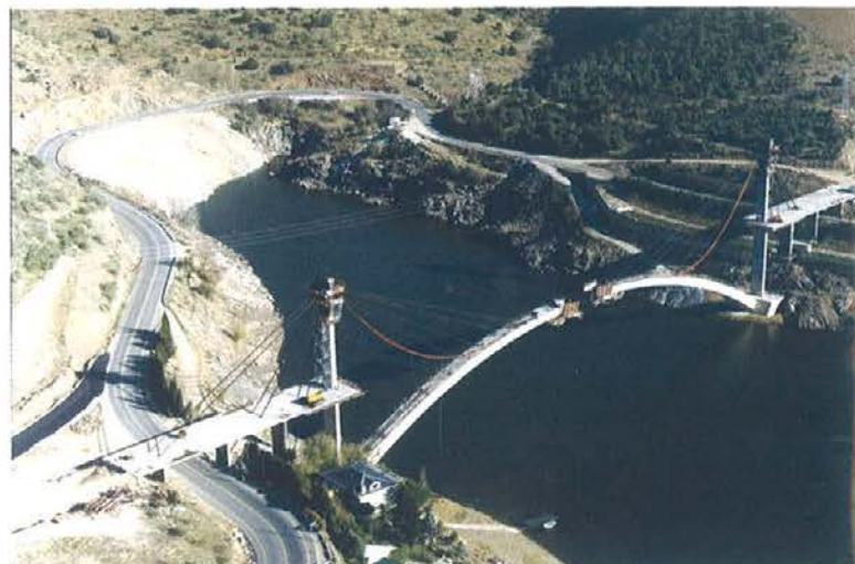
Foto 3. Vistas del arco durante procedimiento constructivo. Picture 3 Views of the arch during the construction procedure.
