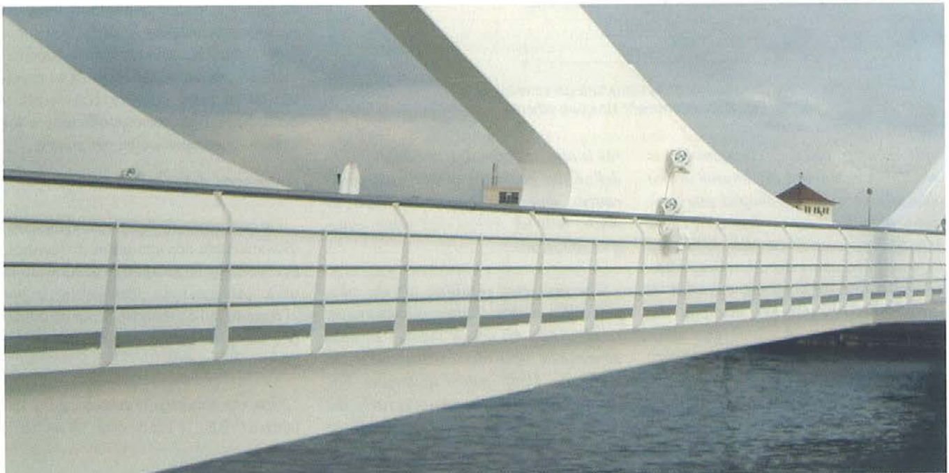
Fig. 6. Vista de la acera. Fig. 6. A view of the pedestrian foot walk.
