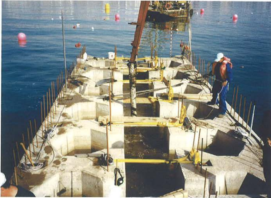
Fig. 16: Hormigonado muro muelle. Fig. 16. Concreting the quays walls.
