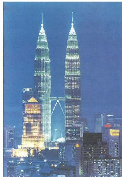
Figura 5. Torres Petronas, Kuala Lumpur.
