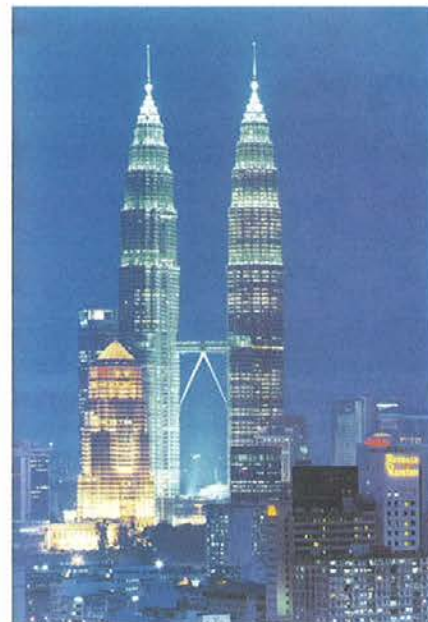
Figura 5. Torres Petronas, Kuala Lumpur.
