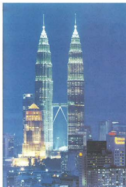
Figura 5. Torres Petronas, Kuala Lumpur.
