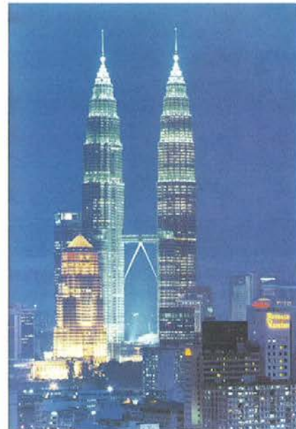
Figura 5. Torres Petronas, Kuala Lumpur.
