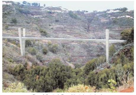
Figura 6. Puente de Teror. Atirantado extradosado. Figure 6. Teror Bridge. Extradosed cable stayed bridge.
