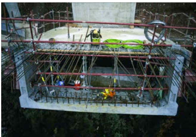
Figura 3. Vista frontal por las dovelas del arco. Figure 3. Front view of segments of the arch.
