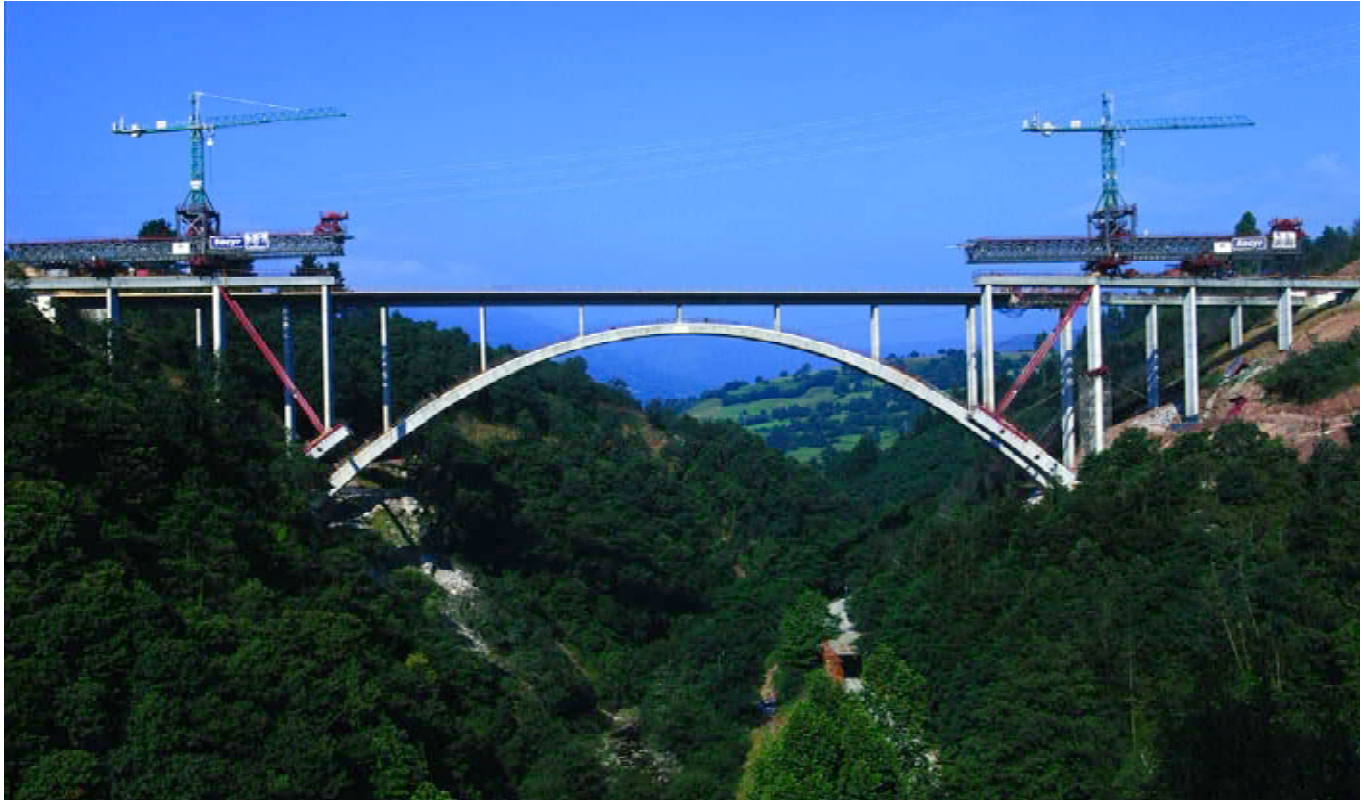
Figura 16. Alzado general del puente durante la construcción. Figure 16. General elevation of the bridge during construction.
