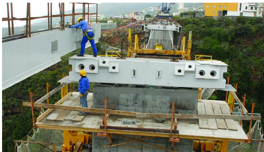
Figura 15. Riostra de pila. Figure 15. Column bracing.
