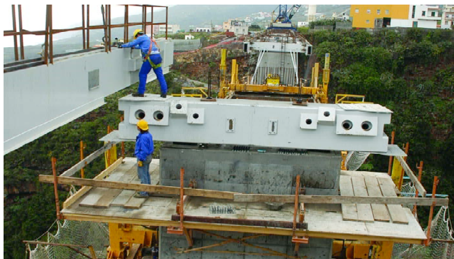
Figura 15. Riostra de pila. Figure 15. Column bracing.
