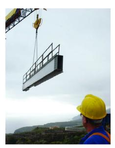
Figura 14. Montaje viga longitudinal. Figure 14. Longitudinal beam assembly.
