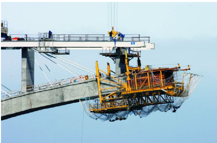
Figura 11. Diagonales auxiliares. Figure 11. Auxiliary diagonals.
