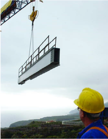
Figura 14. Montaje viga longitudinal. Figure 14. Longitudinal beam assembly.
