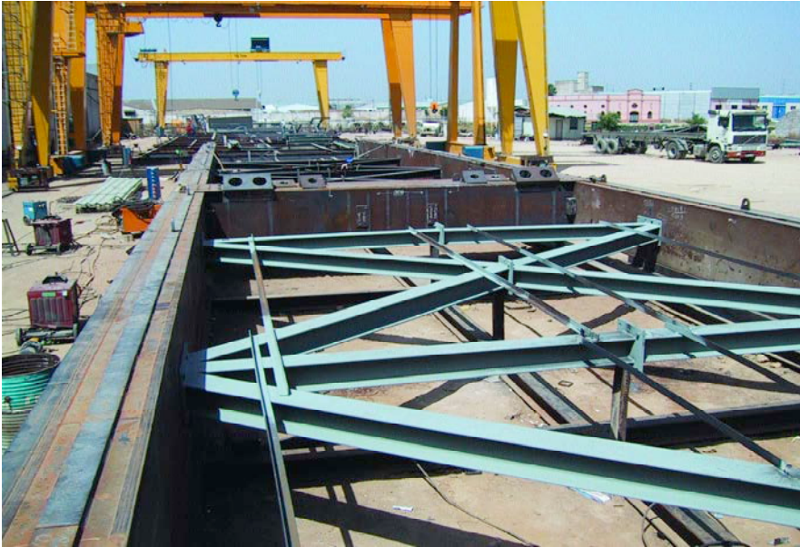
Figura 16. Arriostramiento horizontal. Figure 16. Cross bracing.
