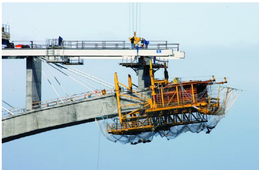
Figura 11. Diagonales auxiliares. Figure 11. Auxiliary diagonals.
