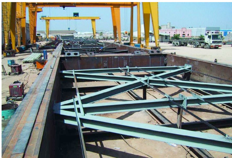
Figura 16. Arriostramiento horizontal. Figure 16. Cross bracing.
