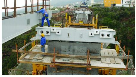
Figura 15. Riostra de pila. *Figure 15. Column bracing.*
