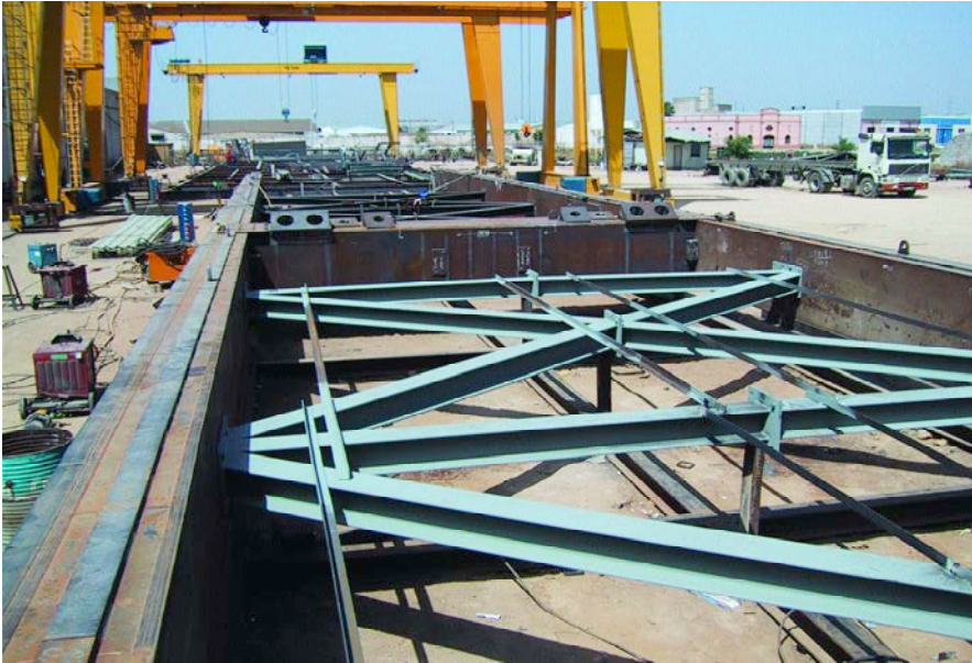
Figura 16. Arriostramiento horizontal. Figure 16. Cross bracing.
