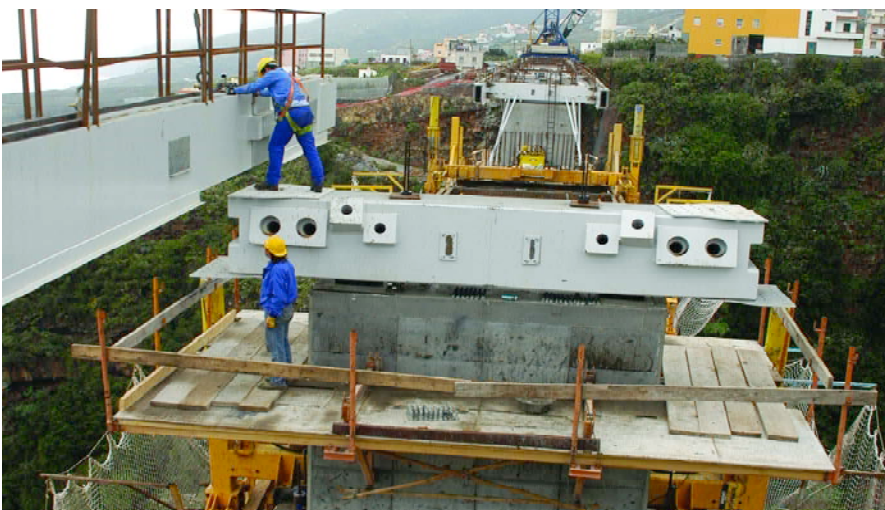
Figura 15. Riostra de pila. Figure 15. Column bracing.
