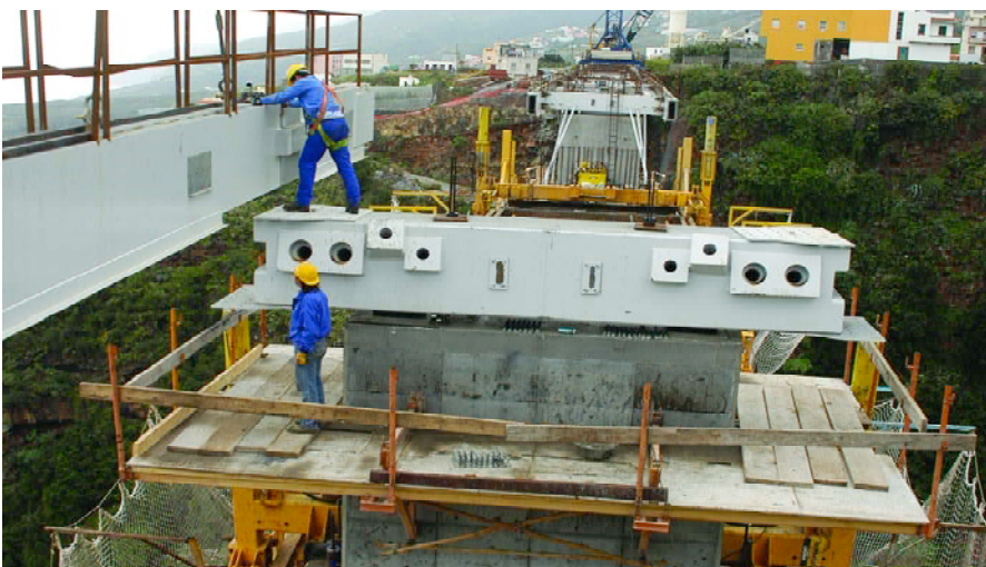
Figura 15. Riostra de pila. Figure 15. Column bracing.
