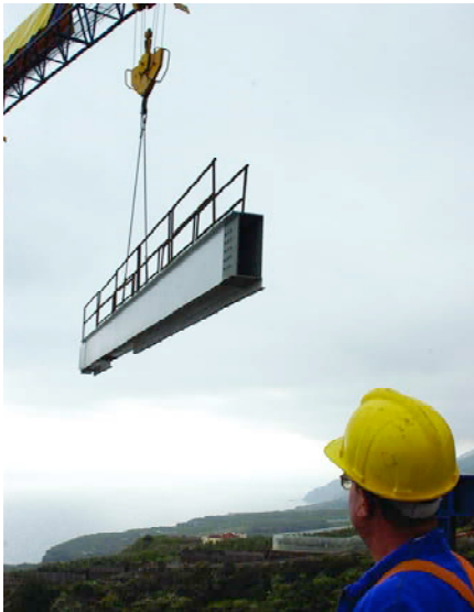
Figura 14. Montaje viga longitudinal. Figure 14. Longitudinal beam assembly.
