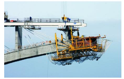
Figura 11. Diagonales auxiliares. Figure 11. Auxiliary diagonals.
