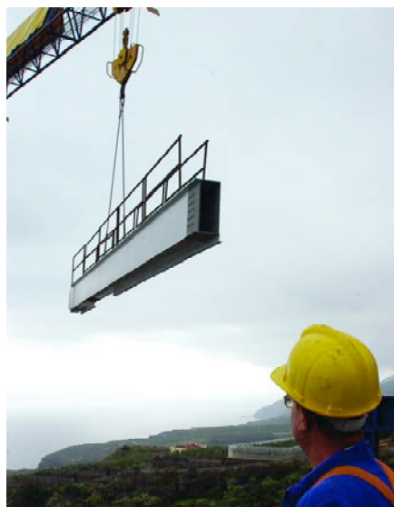
Figura 14. Montaje viga longitudinal. Figure 14. Longitudinal beam assembly.
