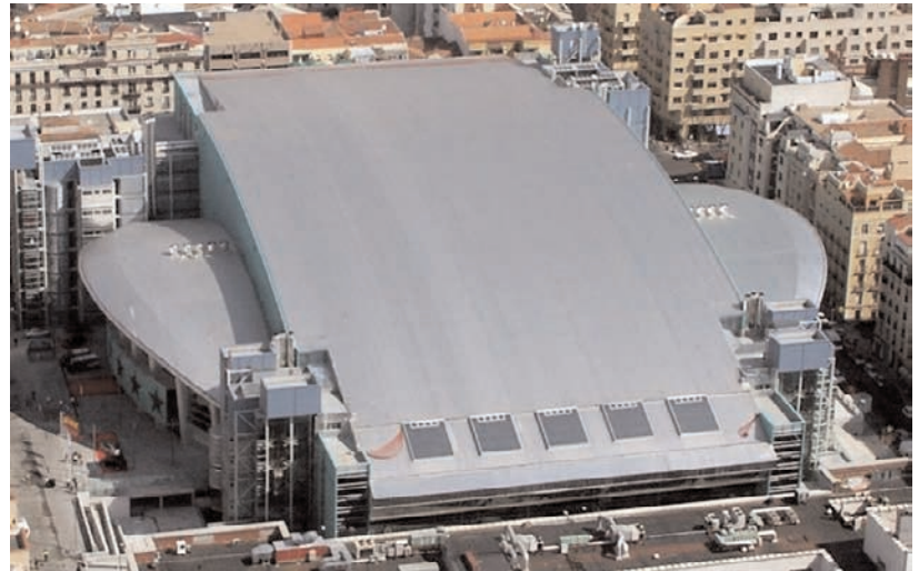
Figura 2. Vista general. Figure 2. General view.
