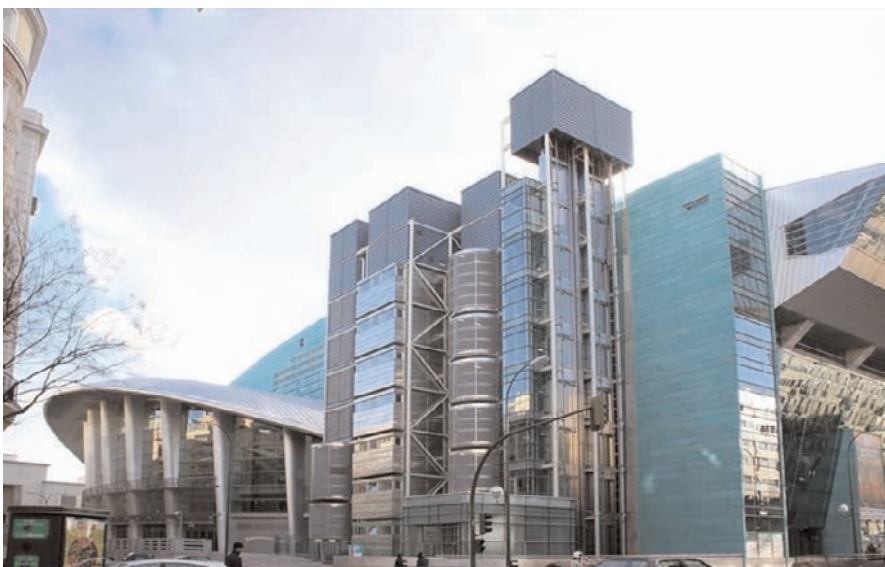
Fig. 18. Torres de Servicios. Figure 18. Service tower.
