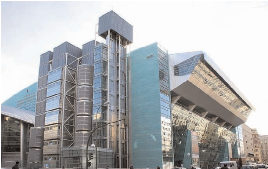
Fig. 26. Fachada del Palacio de Deportes. Figure 26. Façade of sports halls.
