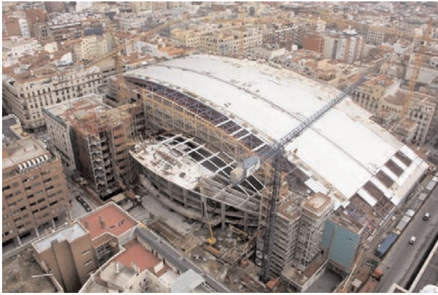
Figuras 10 y 11. Vista exterior e interior de tímpano Figures 10 and 11. External and internal view of the spandrel truss.
