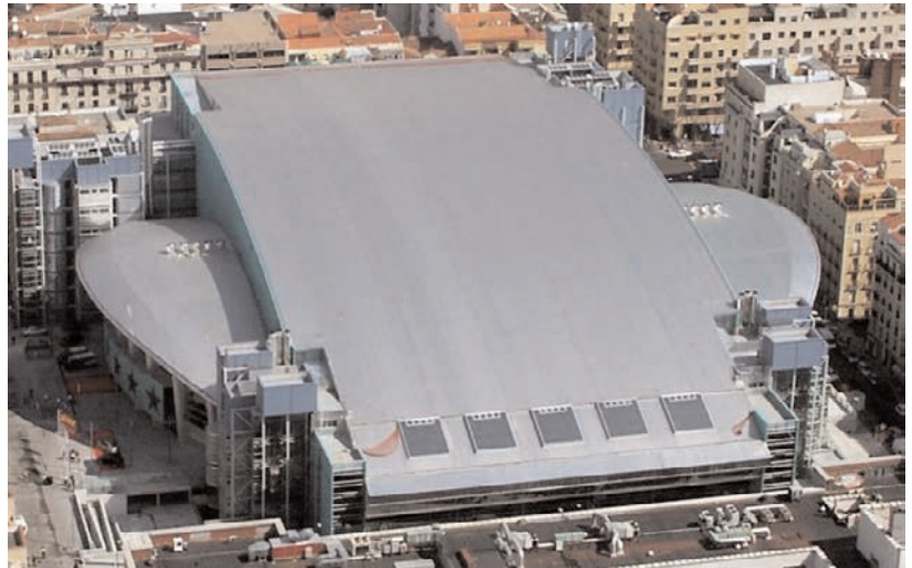
Figura 2. Vista general. Figure 2. General view.
