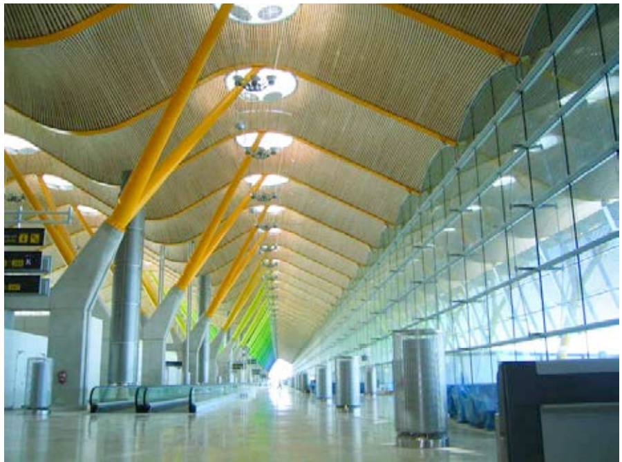
Figura 18. Dique de Terminal, con fachada acristalada. Figure 18. Pier at Terminal Building, with glazed façade.
