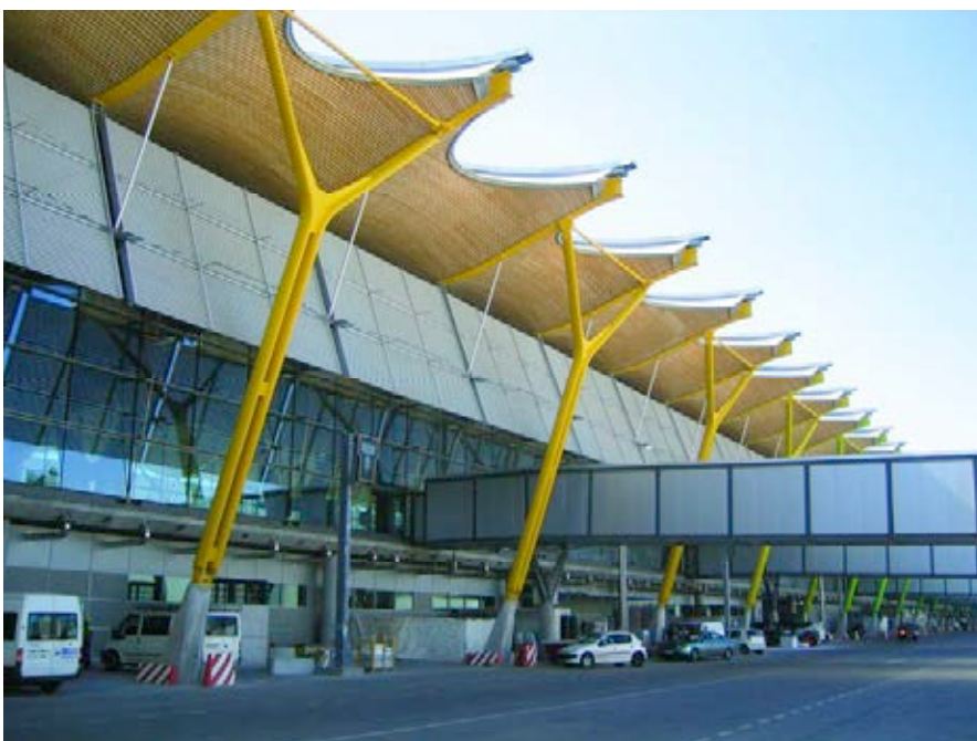
Figura 16. Bambú en los aleros exteriores. Figure 16. Bamboo placed at outside eaves.
