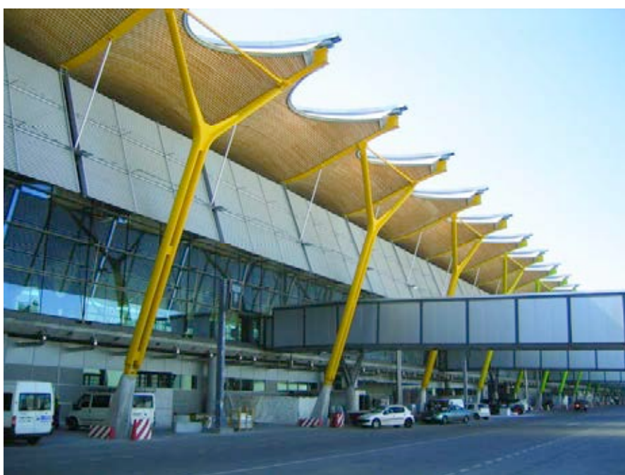
Figura 16. Bambú en los aleros exteriores. Figure 16. Bamboo placed at outside eaves.
