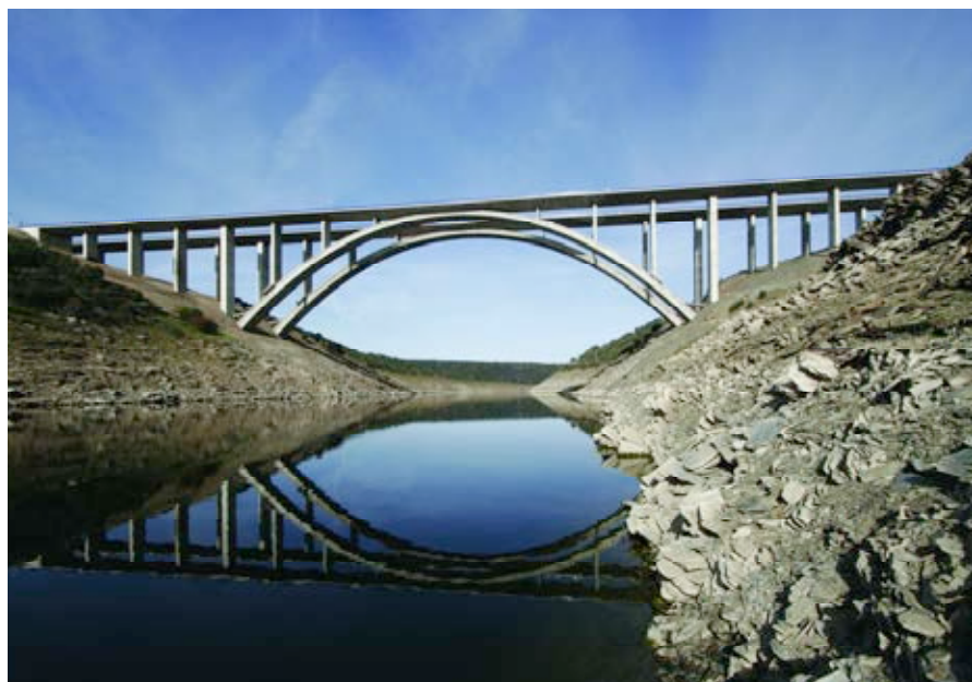
Fig.13. Solución Construida: Vista general. Fig.13. Solution Built: General view.
