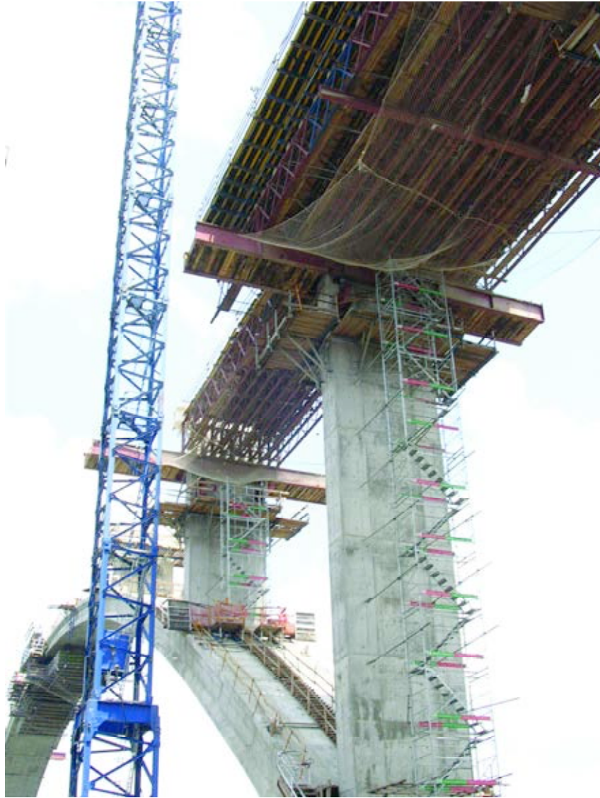
Fig.18. Ejecución del tablero mediante autocimbra. Fig.18. Building the deck with scaffolding truss.
