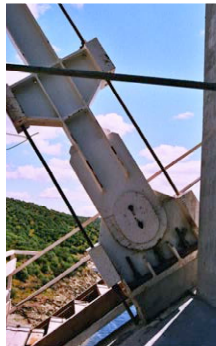
Fig.42. Detalle de tesado de diagonal rígida. Fig.42. Detail of rigid diagonal tensioning.
