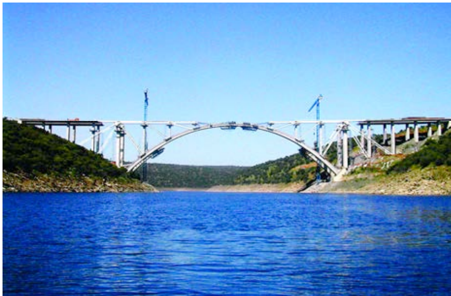
Fig.32. Apertura en clave. Fig.32. Crown opening.
