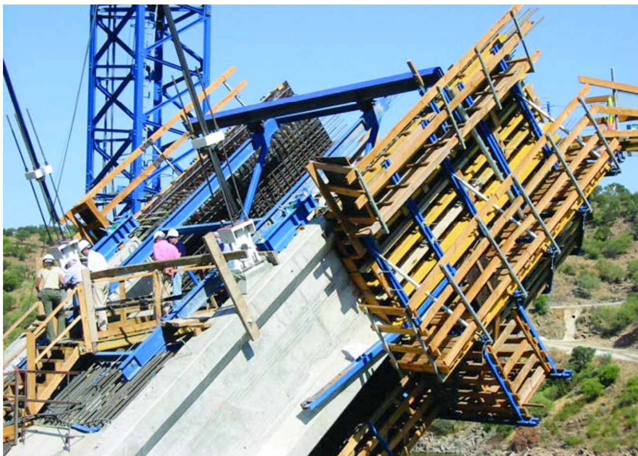
Fig.33. Carro de avance en voladizo para el arco, con tirantes auxiliares. Fig.33. Cantilever advancing carriage for the arch, with auxiliary stays.
