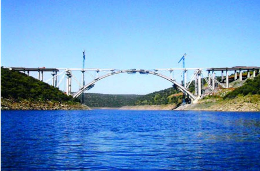
Fig.32. Apertura en clave. Fig.32. Crown opening.
