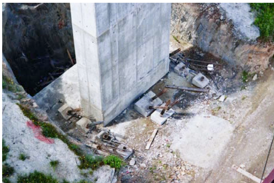
Fig.31. Anclaje de pila 8 al terreno. Fig.31. Anchoring of pier 8 to the ground.
