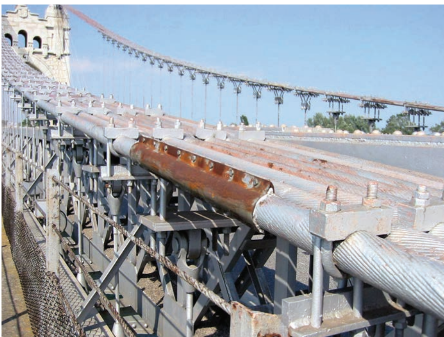
Figura 17. Cables reparados en 1972. Figure 17. Cables repaired in 1972.
