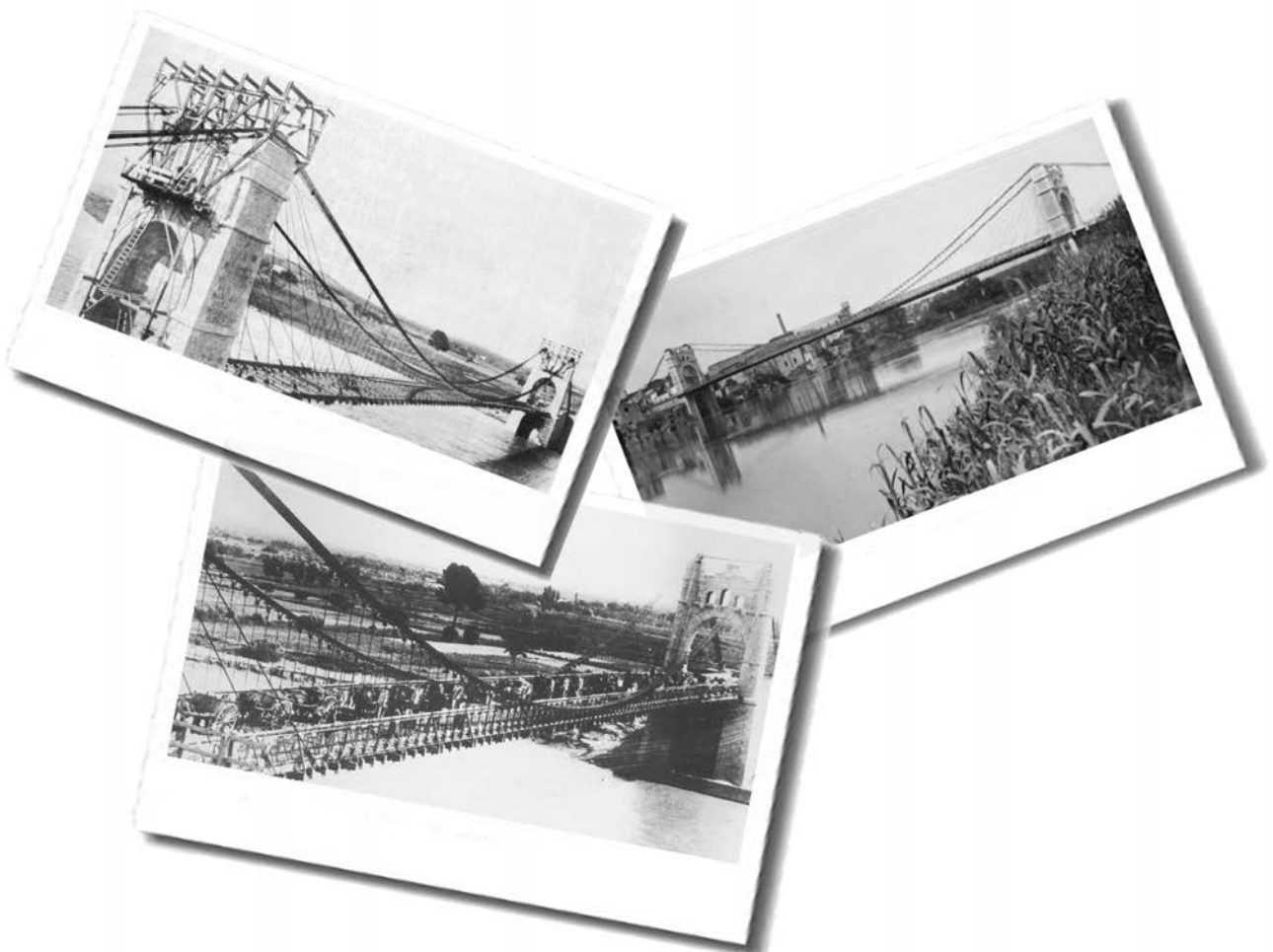
Figura 15. El puente con su aspecto original. Figure 15. The bridge with its original appearance.
