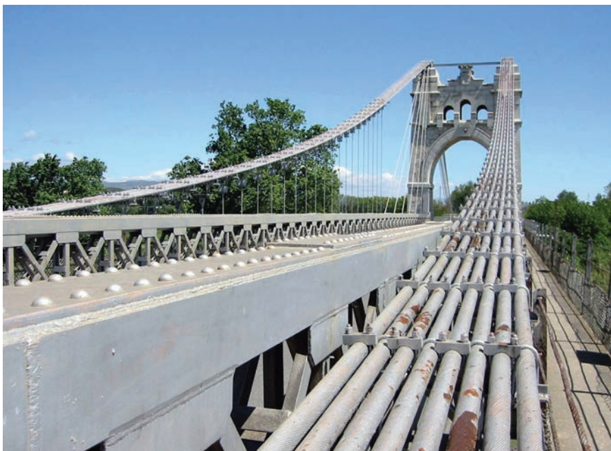
Figura 22. Cables principales. Figure 22. Main cables.
