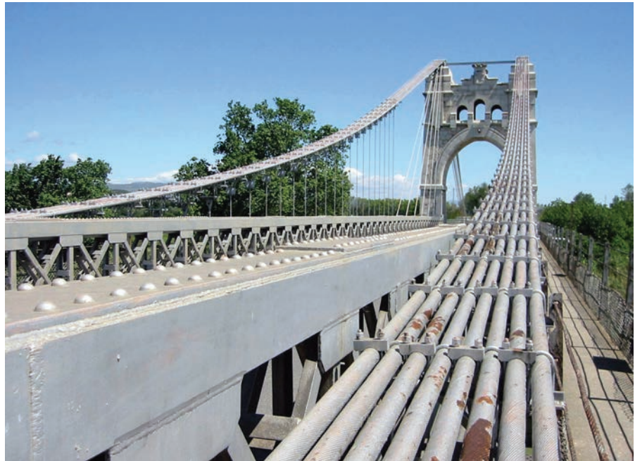
Figura 22. Cables principales. Figure 22. Main cables.
