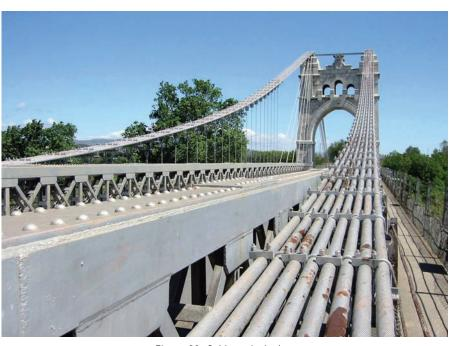
Figura 22. Cables principales. *Figure 22. Main cables.*
