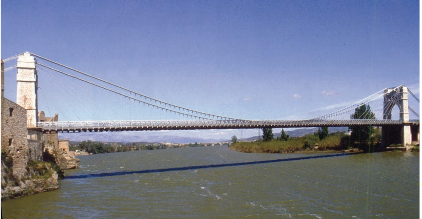
Figura 1. Vista general del puente. Figure 1. General view of the bridge.
