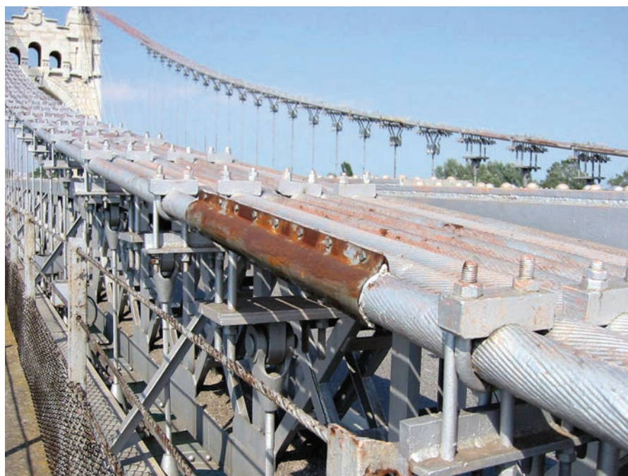
Figura 17. Cables reparados en 1972. Figure 17. Cables repaired in 1972.
