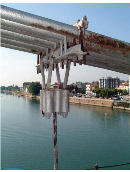
Figura 18. Percha. Figure 18. Hanger.
