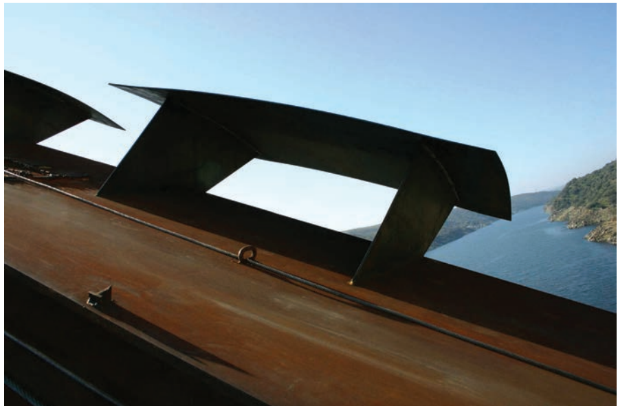
Figura 58. Deflector. Detalle. Figure 58. Guide vane. Detail.
