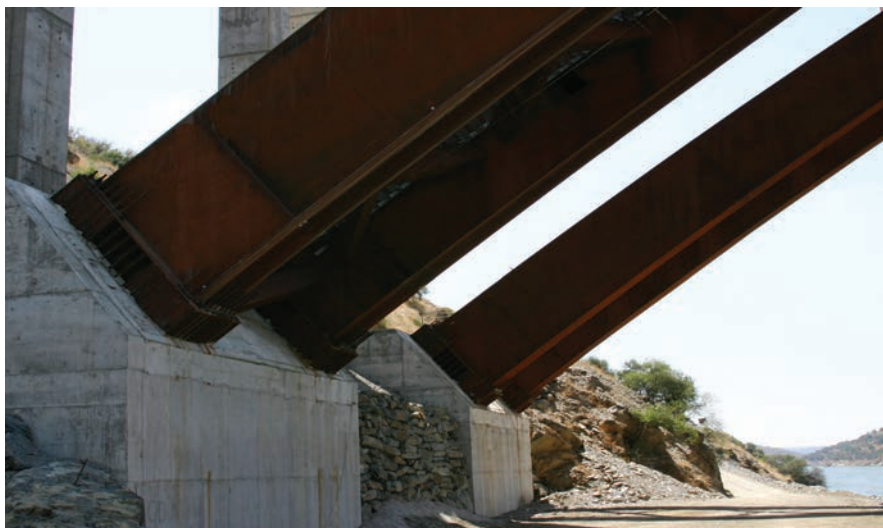
Figura 10. Empotramiento del arco. Figure 10. Arch fixing.
