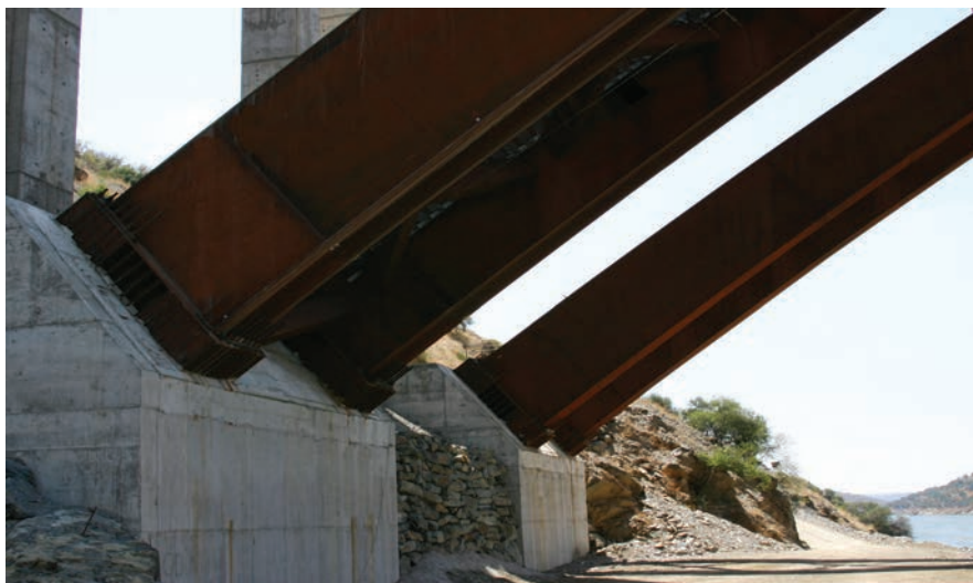
Figura 10. Empotramiento del arco. Figure 10. Arch fixing.
