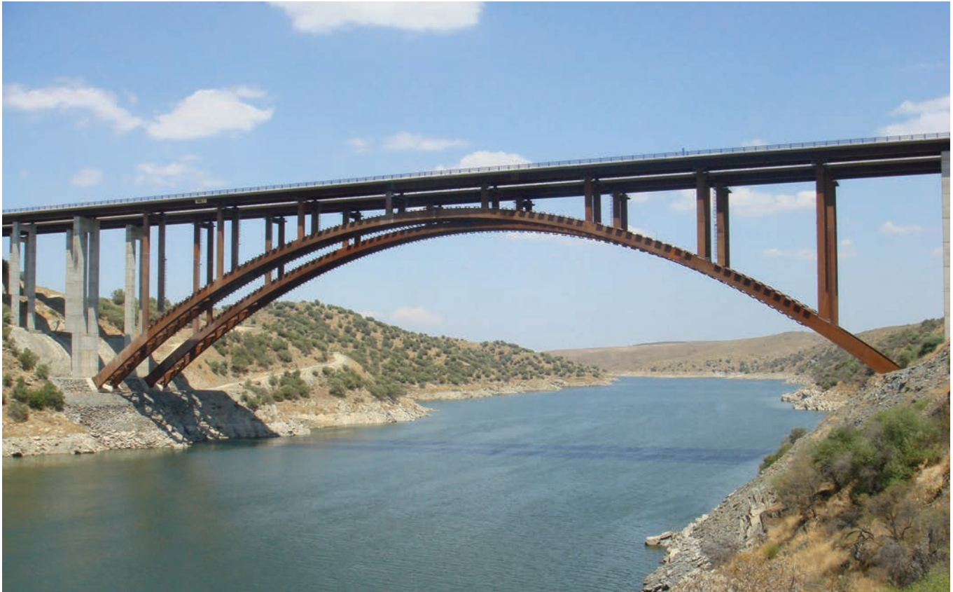
Figura 1. Vista general. Figure 1. General view.
