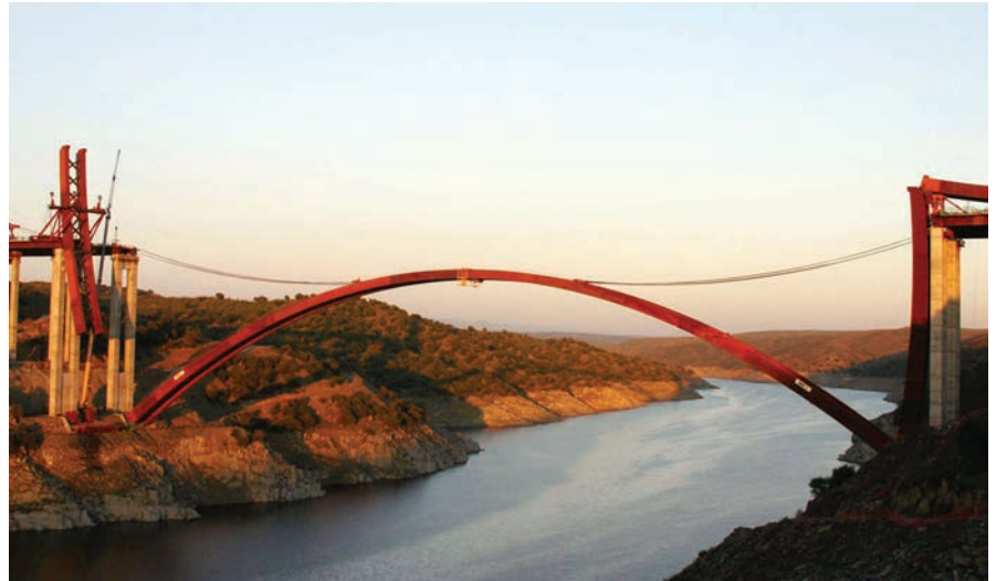
Figura 35. Cierre en clave. Figure 35. Crown closure.
