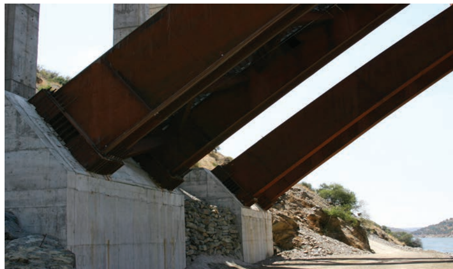
Figura 10. Empotramiento del arco. Figure 10. Arch fixing.
