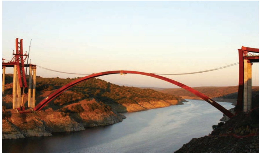
Figura 35. Cierre en clave. Figure 35. Crown closure.
