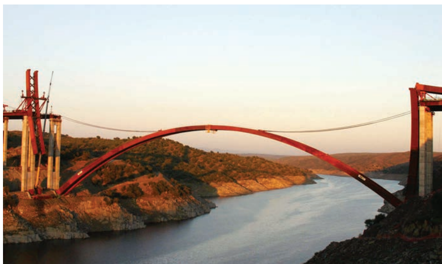
Figura 35. Cierre en clave. Figure 35. Crown closure.
