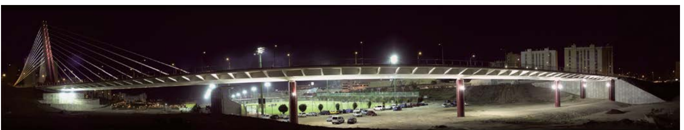
Figura 6. Vista del viaducto iluminado desde el parque Figure 6. View of the illuminated viaduct from the park.
