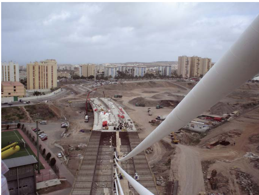
Figura 36. Montaje del tirante 10. Figure 36. Assembly of the tenth stay.
