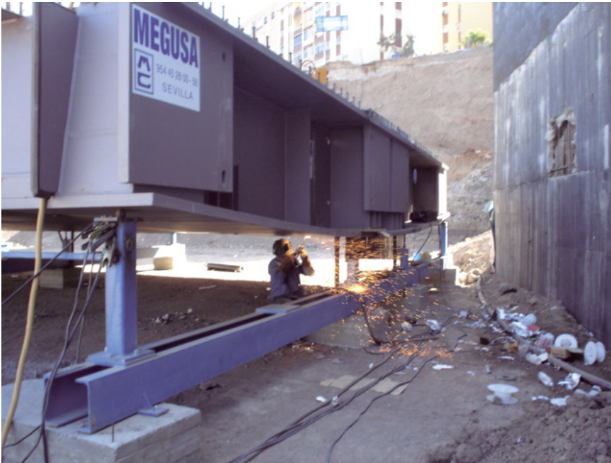
Figura 16. Diafragma de estribo 1. Figure 16. Diaphragm of abutment 1.
