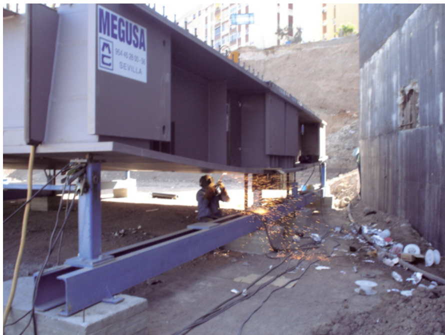
Figura 16. Diafragma de estribo 1. Figure 16. Diaphragm of abutment 1.
