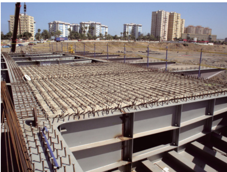
Figura 17. Prelosas en el tablero. Figure 17. Stay-in-place concrete panels on the deck.
