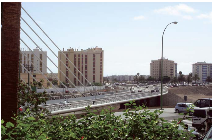
Figura 10. Vista general del viaducto insertado dentro del viario de la ciudad. Figure 10. General view of the viaduct integrated into the road network of the city.
