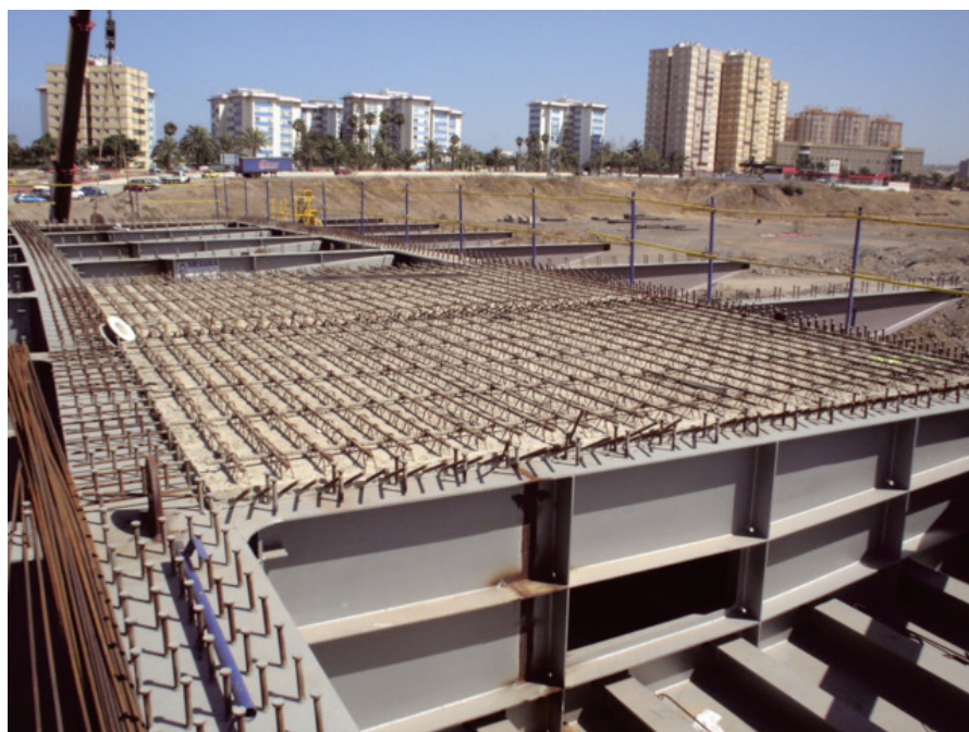
Figura 17. Prelas en el tablero. Figure 17. Stay-in-place concrete panels on the deck.
