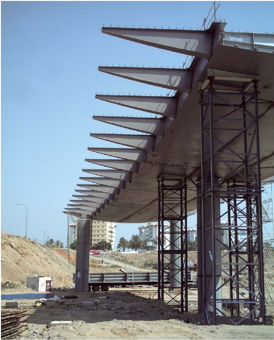
Figura 14. Costillas metálicas Figure 14. Metal ribs.
