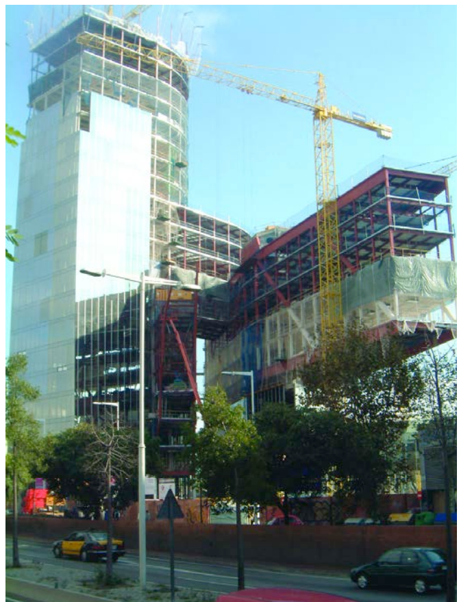
Figura 30. Vista general en fase de terminaciones. Figure 30. General view of finishing work.
