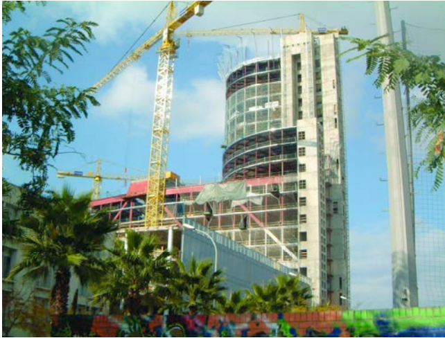
Figura 31. Vista dorsal en fase de cerramiento. Figure 31. Rear view during construction of facings.
