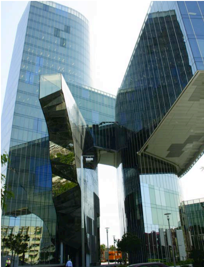
Figura 35. Vista longitudinal del capitel y de la calle interior en el edificio terminado. Figure 35 Longitudinal view of the Capital building and the inner avenue to the finished building.
