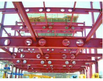
Figura 28. Estructura de vigas de una planta del Portaaviones Figure 28. Beam structure on one floor of the Aircraft-carrier building.
