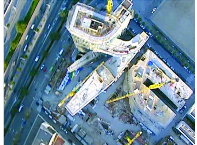
Figura 32. Vista aérea en planta durante la construcción. Figure 32. Aerial view of the site during construction.
