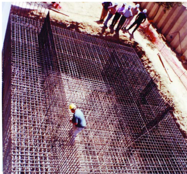
Figura 51. Armado del encepado. Figure 51. Reinforcement of the pile caps.
