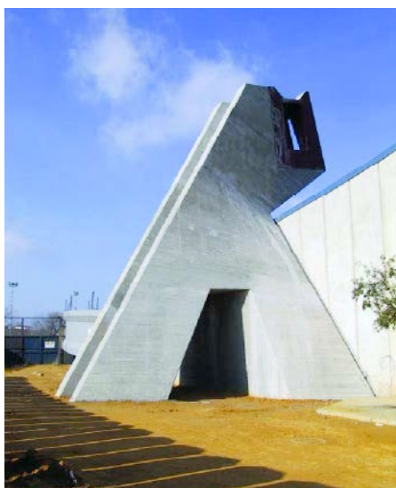
Figura 16. Vista del soporte desde el exterior. Figure 16. View of the support from the outside.
