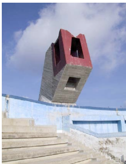
Figura 17. Vista del soporte desde el interior. Figure 17. View of the support from the inside.
