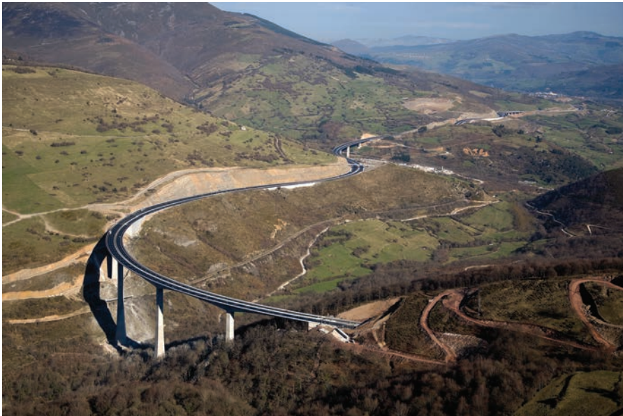
Figura 4. Vista general de la traza de la autovía. Figure 4. General view of the dual carriageway's alignment.
