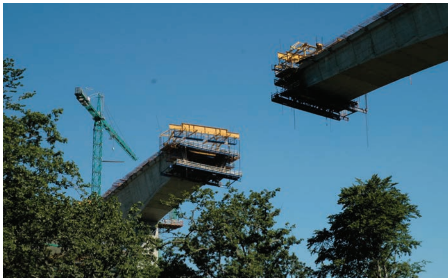
Figura 30. Detalle de carros acercándose en pilas 2 y 3. Figure 30. Detail of travellers approaching each other at piers 2 and 3.
