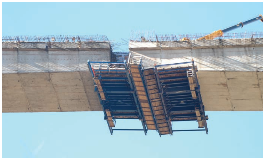
Figura 31. Vista inferior de encofrado de dovela de cierre Figure 31. Underneath view of the connection segment's formwork.
