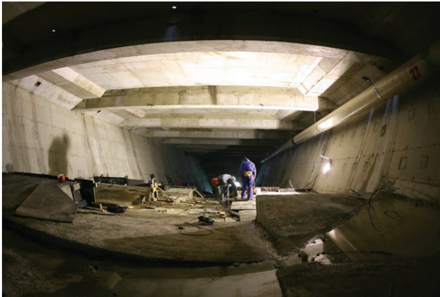
Figura 17. Detalle de interior de tablero. Figure 17. Detail of the deck's interior.
