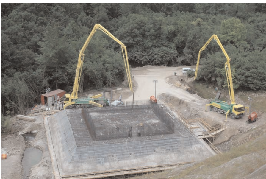
Figura 8. Hormigonado de encepado de pila 2. Figure 8. Concreting pier 2's capping.
