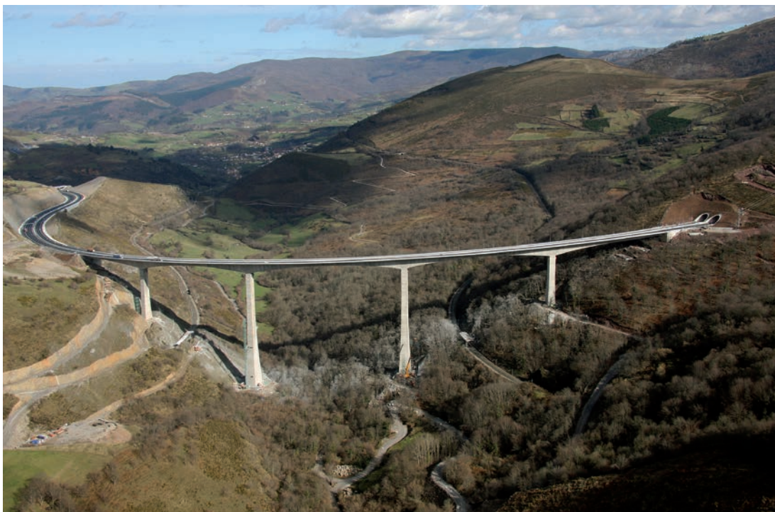
Figura 43. Vista general del Viaducto. Figure 43. General view of the viaduct.
