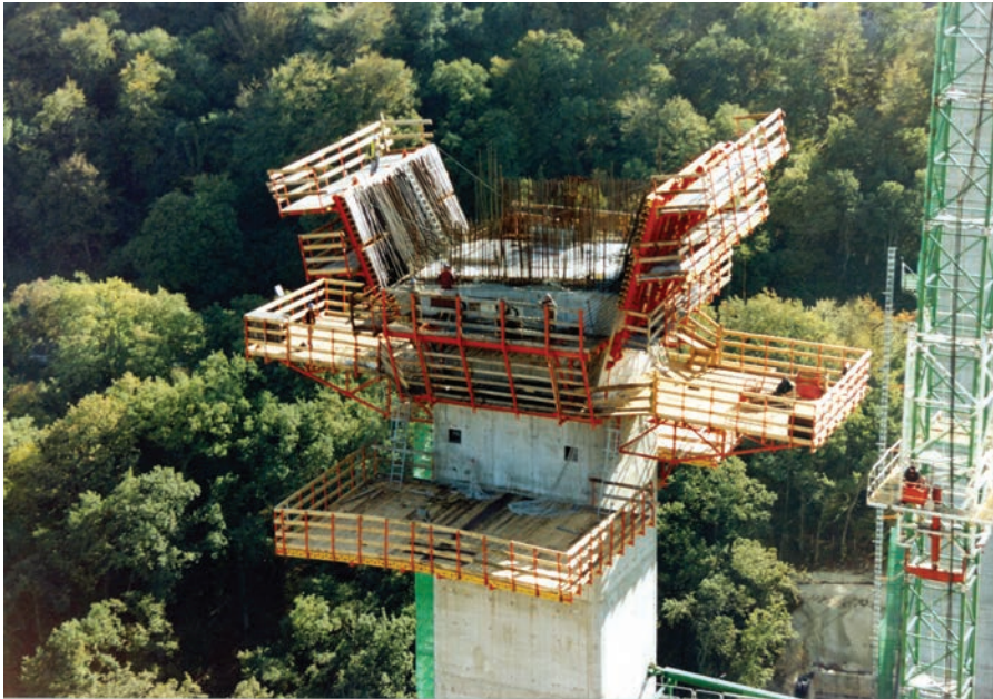
Figura 25. Ejecución de la dovela "0". Figure 25. Execution of the "0" segment.
