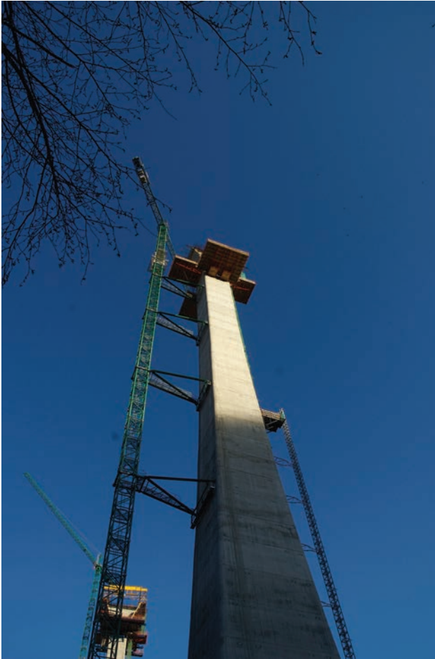
Figura 11. Vista inferior de pila 2. Figure 11. Underneath view of pier 2.
