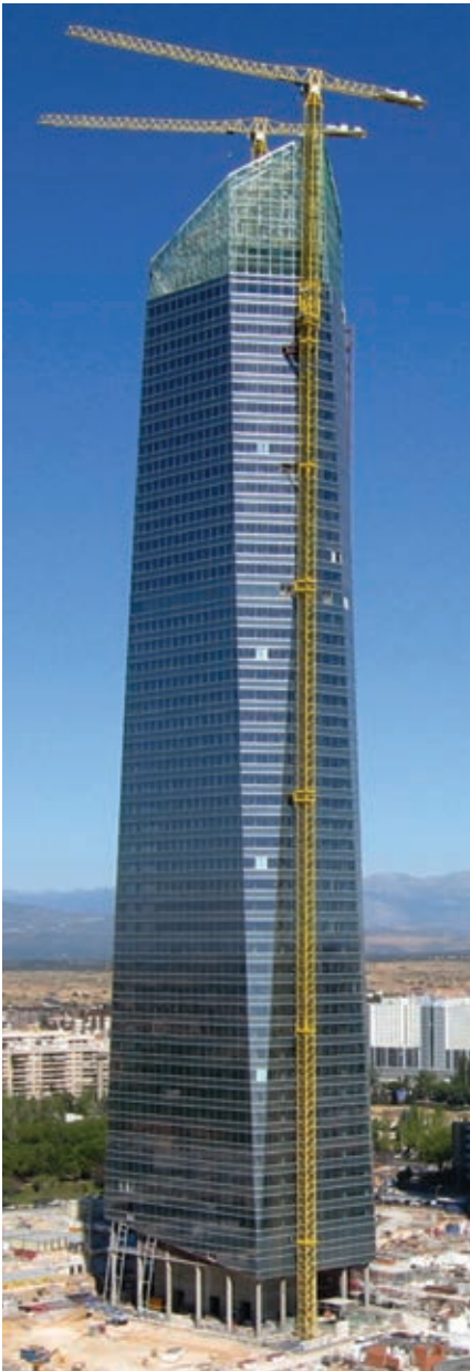
Figura 1. Torre. Vista general. Figure 1. Tower. Overview.
