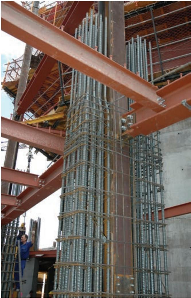
erate bracing for the cantilevers of the supports.
