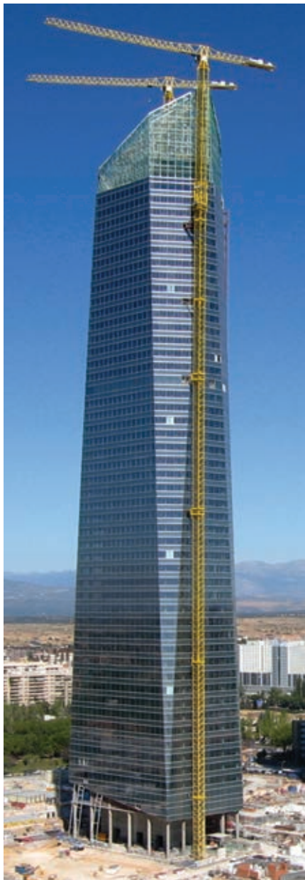
Figura 1. Torre. Vista general. Figure 1. Tower. Overview.
