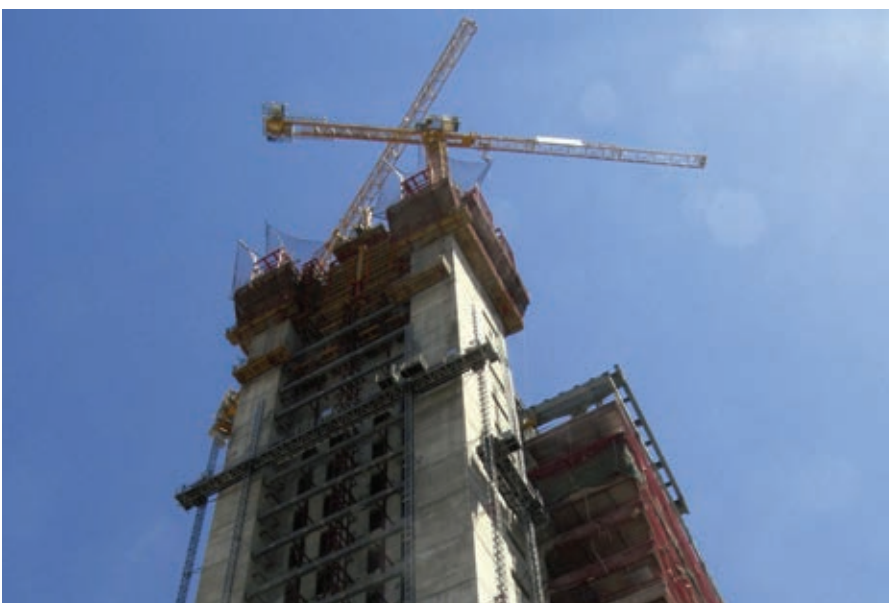
Figura 6. Plataformas eléctricas de fachada. Figure 6. Electrically powered facade platforms.
