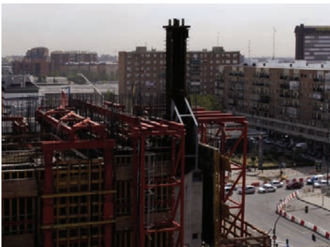
Figura 20. Pilar embebido y cerchas principales. Figure 20. Embedded column and main trusses.
