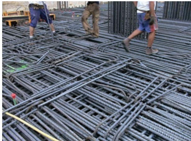
Figura 8. Arranque de soportes de torre y cierre de torretas de cortante. Figure 8. Start of the tower supports and end of the shear turrets.
