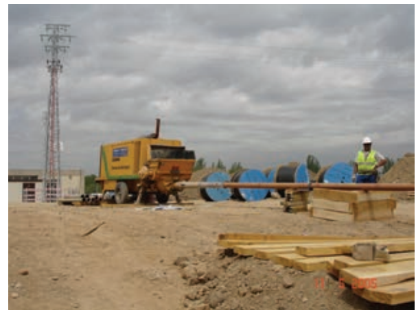
Figura 3. Bombeo de hormigón. Figure 3. Concrete pumping.
