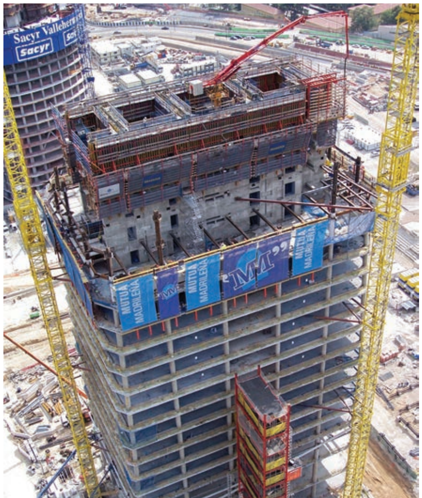
Figura 1. Vista general de grúas y ascensor de obra. Figure 1. General view of cranes and construction hoist.
