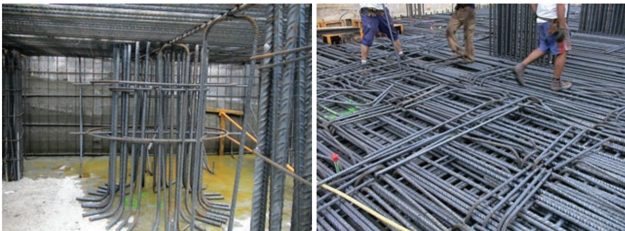
Figura 8. Arranque de soportes de torre y cierre de torretas de cortante. Figure 8. Start of the tower supports and end of the shear turrets.
