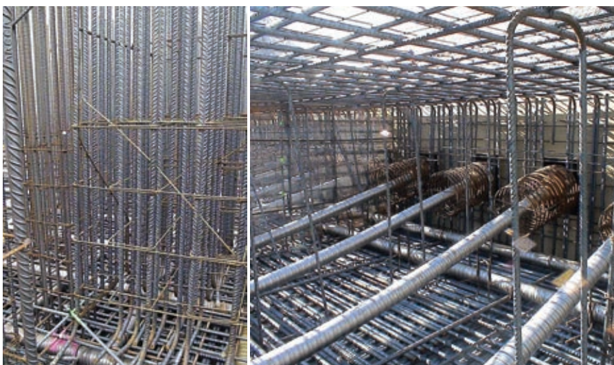
Figura 3. Detalle de arranque de núcleo central y fijación de cabezas al encofrado. Figure 3. Detail of the foot of the central core and attachment of the prestressing heads to the formwork.
