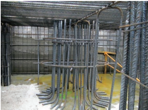
Figura 8. Arranque de soportes de torre y cierre de torretas de cortante. Figure 8. Start of the tower supports and end of the shear turrets.
