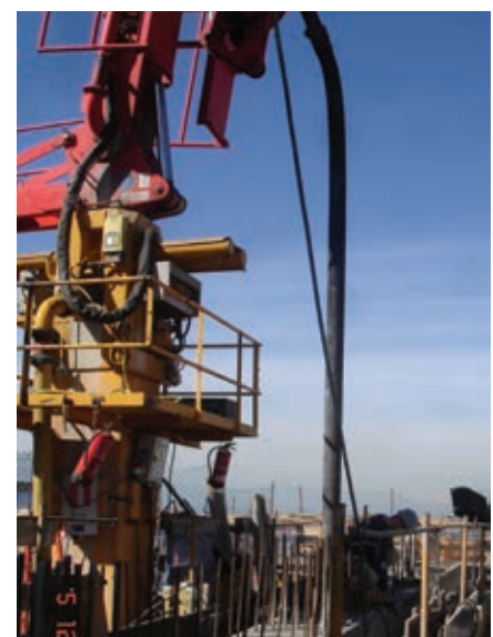
Figura 4. Bombeo de hormigón. Figure 4. Concrete pumping.
