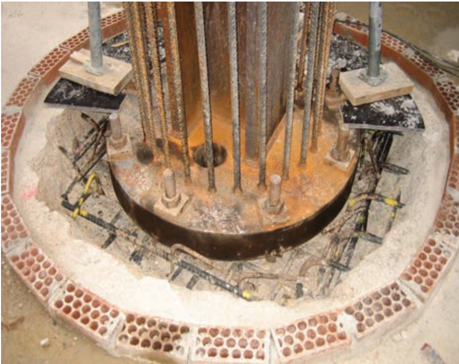
Figura 15. Detalle de la zona a hormigonar bajo placa. Figure 15. Detail of the area to be concreted under the plate.
