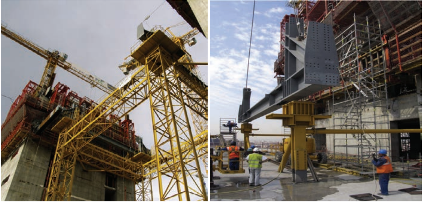
Figura 22. Apeos de cerchas en planta PT1 (izda.) y en PT 2 y PT3 (dcha.). Figure 22. Supports for PT1 (left) and PT2 and PT3 (right) trusses.
