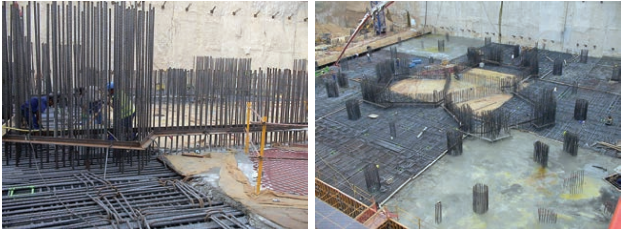
Figura 9. Plantilla de colocación de armado de núcleo y vista general del hormigonado de la segunda tongada de losa. Figure 9. Mould for the installation of the core reinforcement and general view of the concreting of the second concrete lift of the slab.
