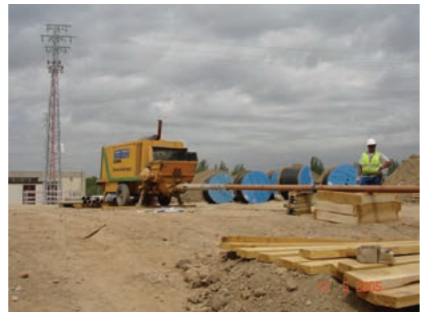
Figura 3. Bombeo de hormigón. Figure 3. Concrete pumping.
