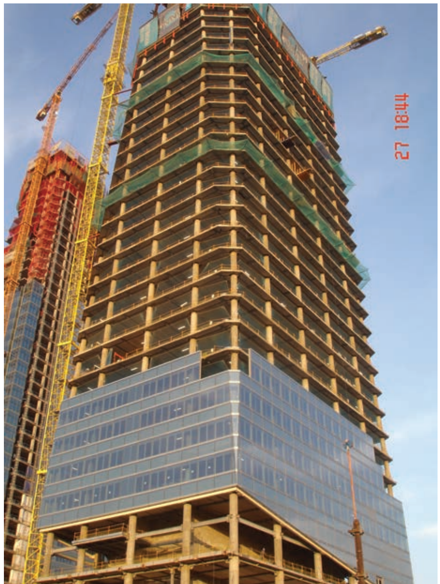
Figura 18. Muro cortina parcialmente instalado, Figure 18. Partially installed curtain wall.
