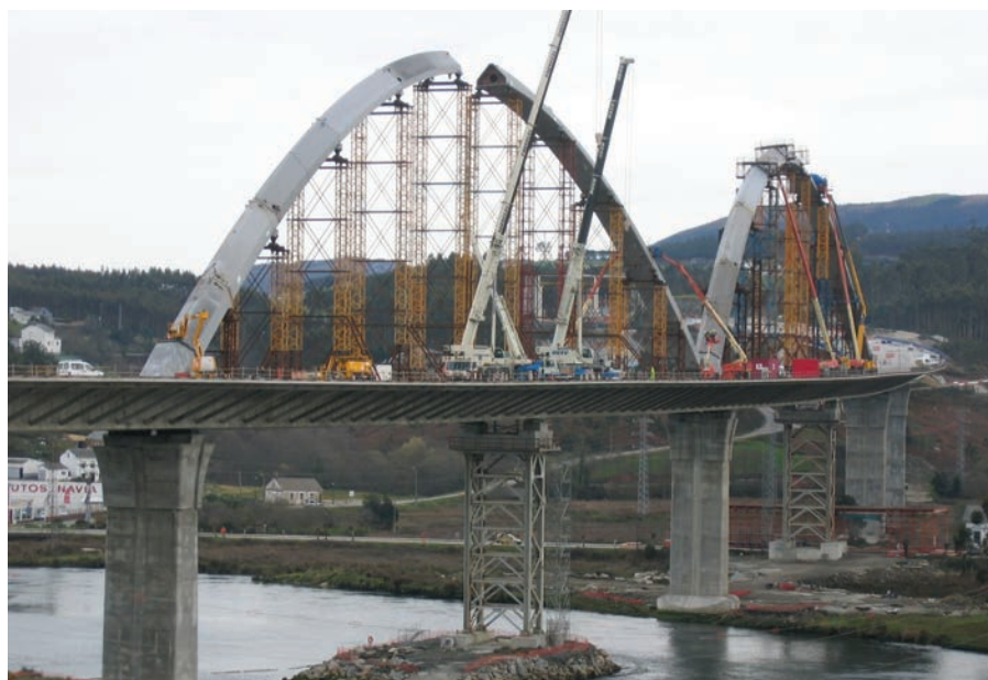
Figura 19. Montaje de arcos. Figure 19. Arch assembly.
