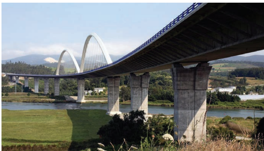
Figura 1. Vista General. Figure 1. Overview.
