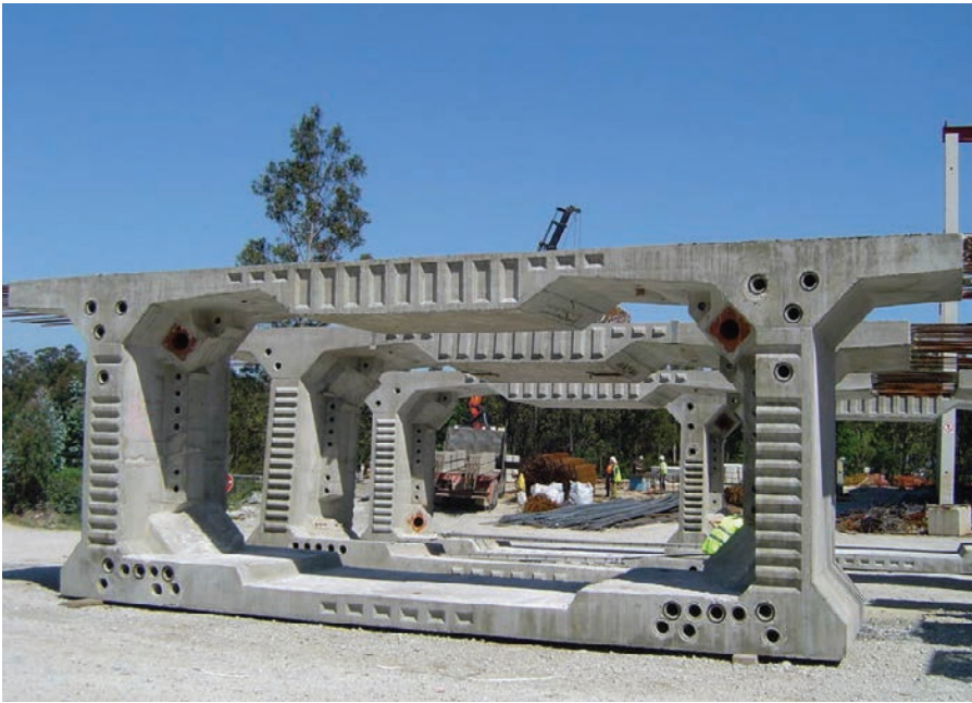
Figura 9. Dovela vanos en arco. Figure 9. Arch span segments.
