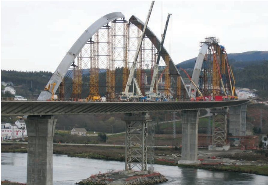
Figura 19. Montaje de arcos. Figure 19. Arch assembly.
