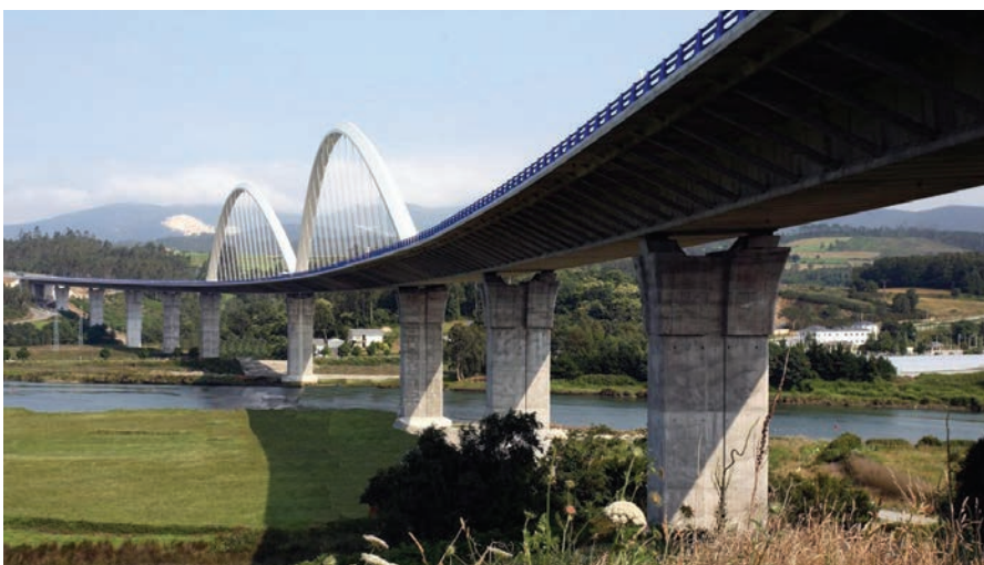
Figura 1. Vista General. Figure 1. Overview.
