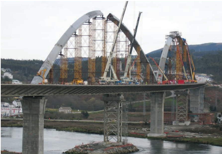
Figura 19. Montaje de arcos. Figure 19. Arch assembly.
