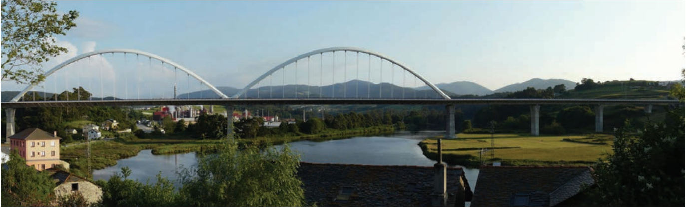
Figura 2. Vista de la ría de Navia. Figure 2. View of the Navia Estuary.
