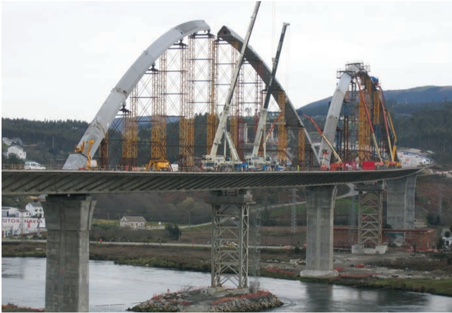
Figura 19. Montaje de arcos. Figure 19. Arch assembly.
