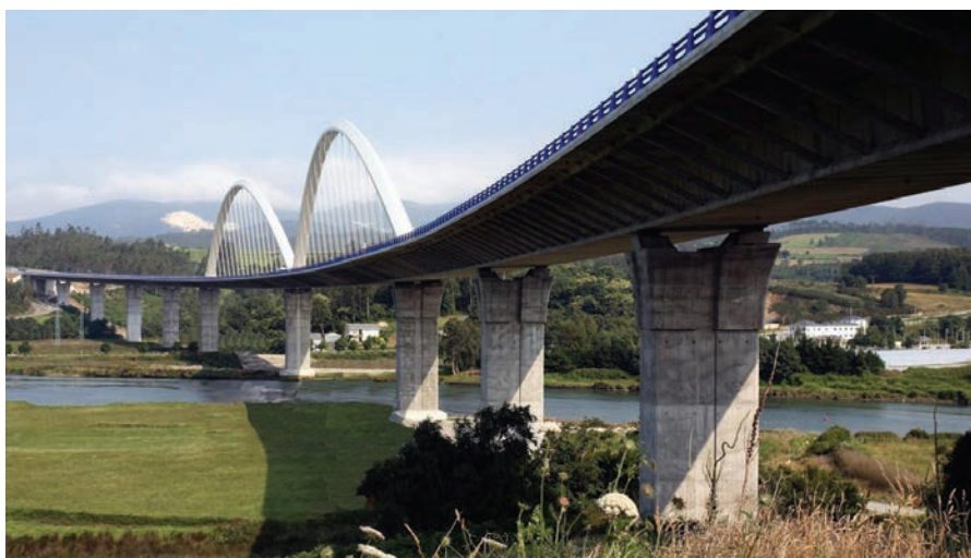
Figura 1. Vista General. Figure 1. Overview.
