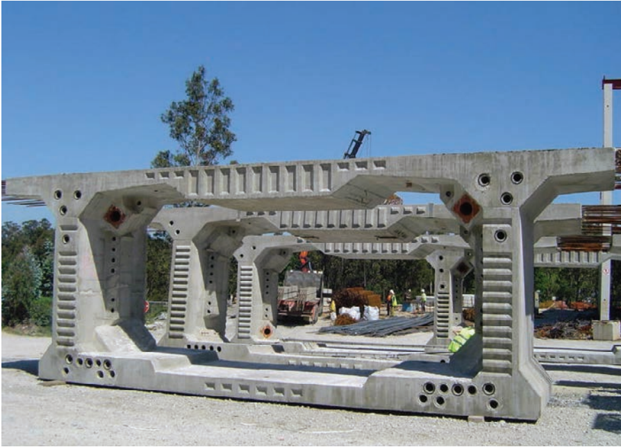
Figura 9. Dovela vanos en arco. Figure 9. Arch span segments.
