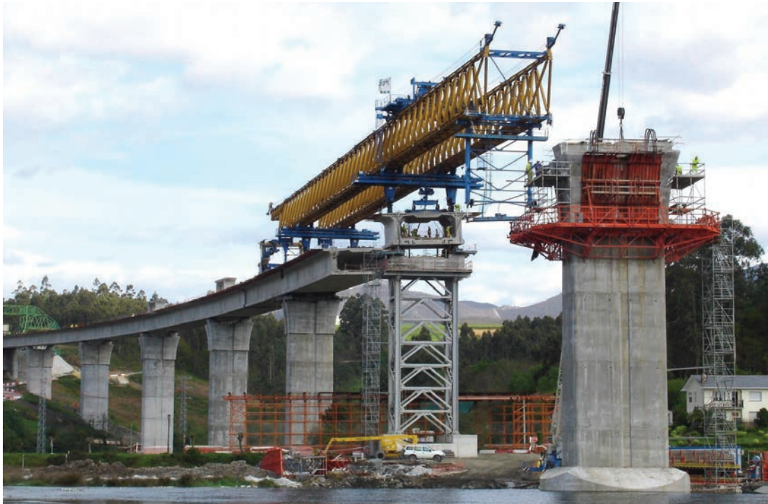
Figura 17. Montaje de dovelas. Figure 17. Segment assembly.
