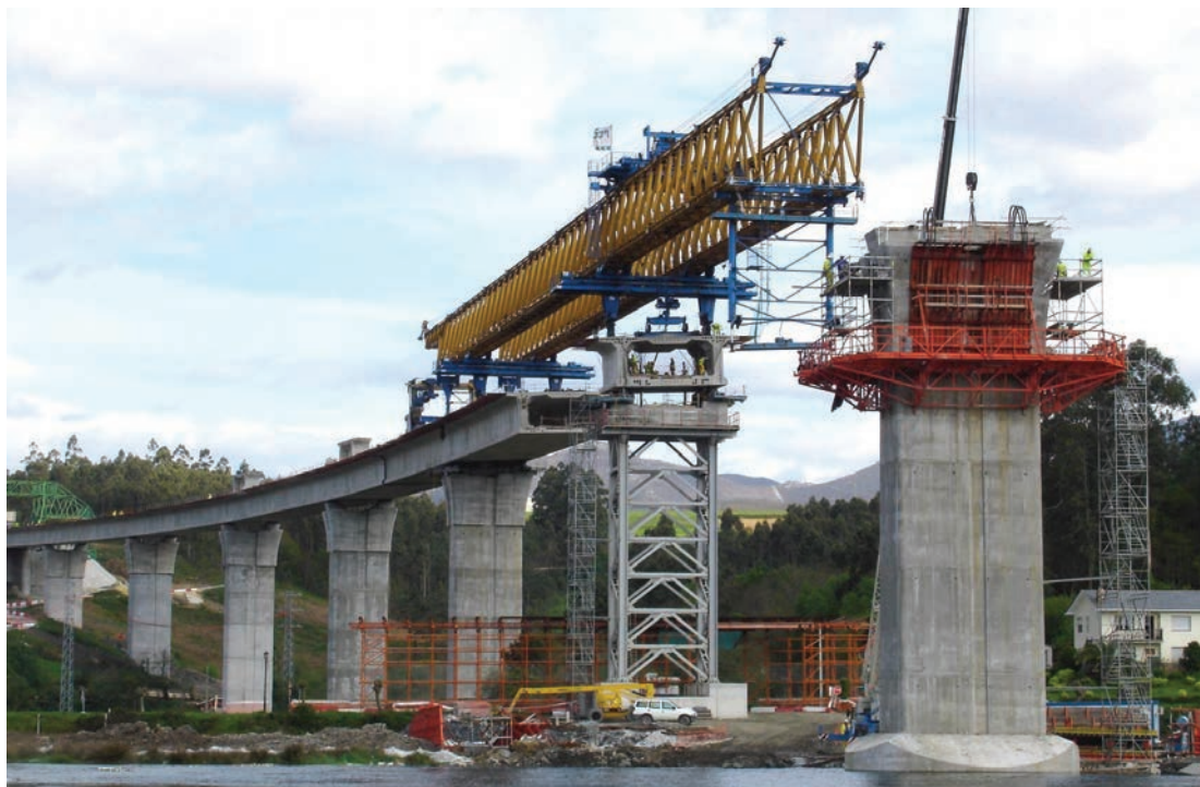
Figura 17. Montaje de dovelas. Figure 17. Segment assembly.
