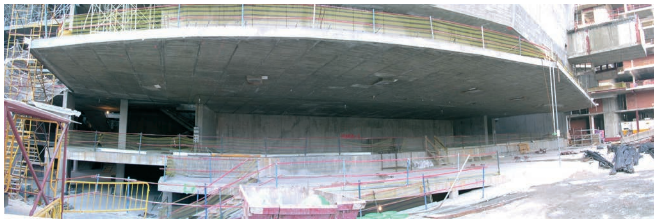
Figura 11. Vista inferior de la gran losa volada del Teatro Principal. Figure 11. Main Theatre cantilever access slab lower view.
