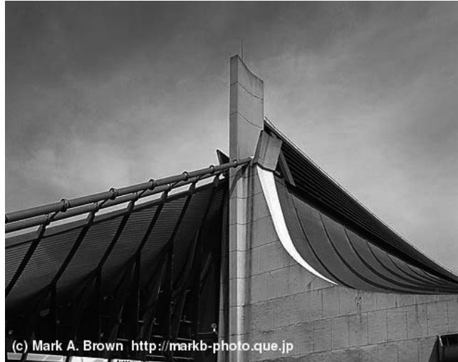
Kenzo Tange. Pabellón Principal . Tokyo, 1964.
