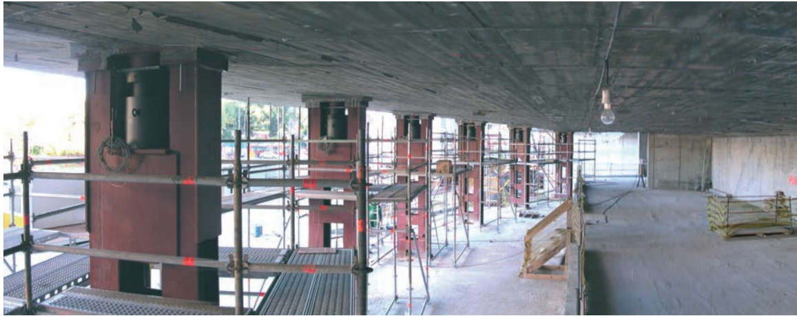
Figura 38. Apeos del Teatro principal con los gatos de desapeo colocados. Figure 38. Hydraulic jacks on the temporary supports of the Main Theatre.
