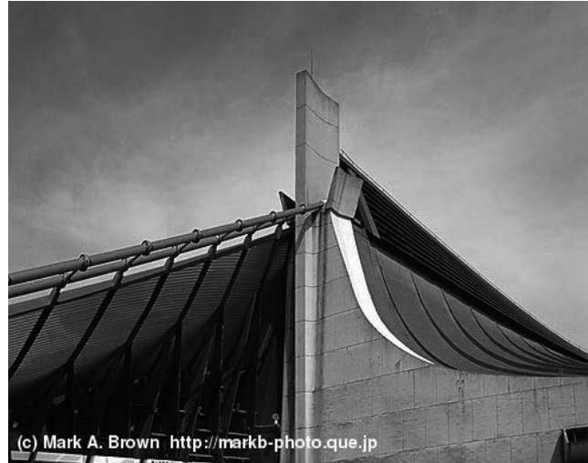
Kenzo Tange. Pabellón Principal . Tokyo, 1964.
