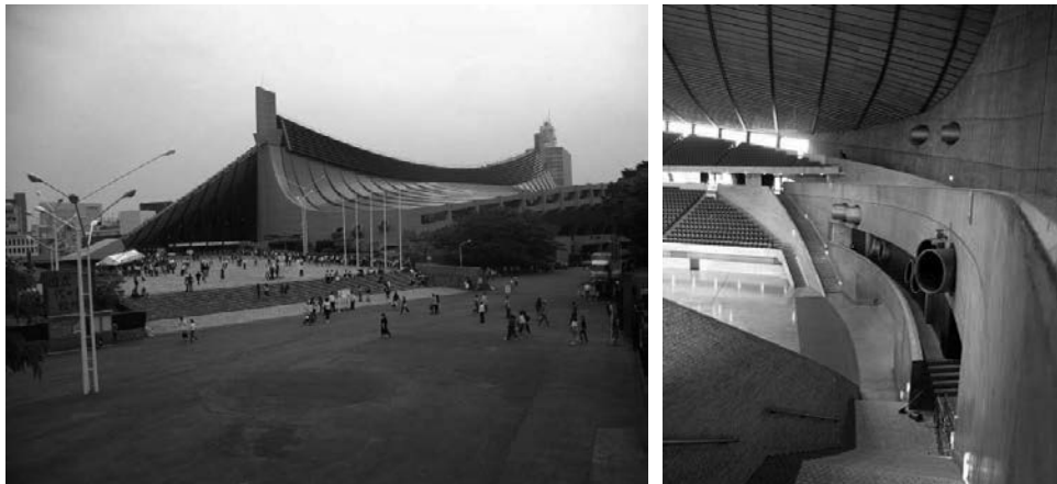
Kenzo Tange. Pabellón Principal . Tokyo, 1964.
