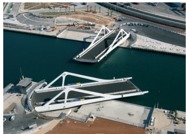
Figura 10. Movimiento de la hoja. Tableros isostáticos. Figure 10. Leaf movement. Statically determinate leaves.
