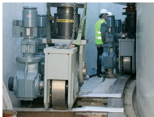
Figura 38. Colocación de carretones Figure 38. Traction wheel installation.
