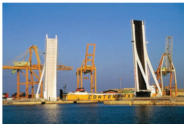
Figura 3. Puente basculante original. Figure 3. Original bascule bridge
