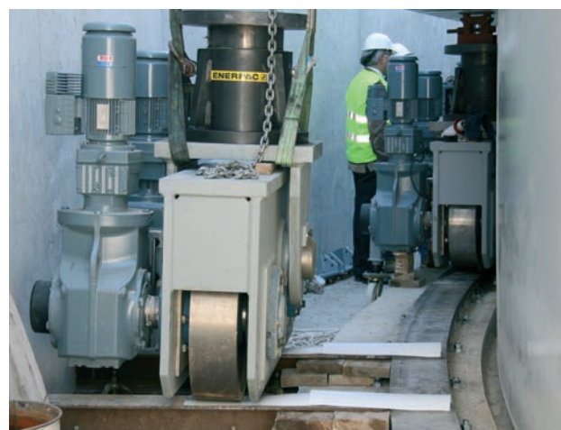
Figura 38. Colocación de carretones Figure 38. Traction wheel installation.
