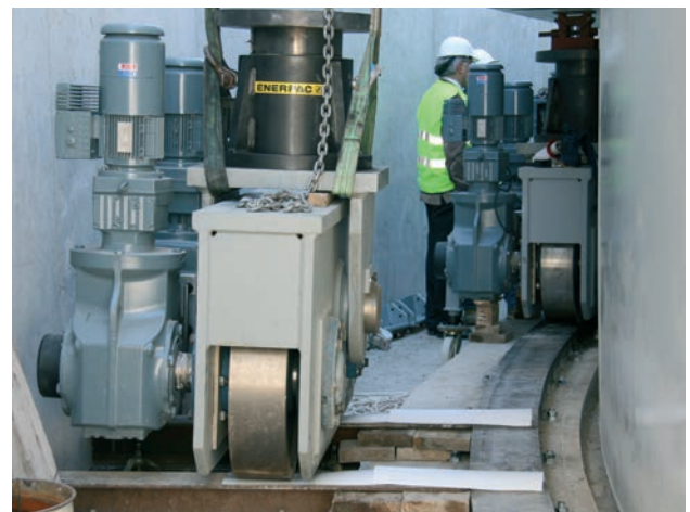
Figura 38. Colocación de carretones Figure 38. Traction wheel installation.
