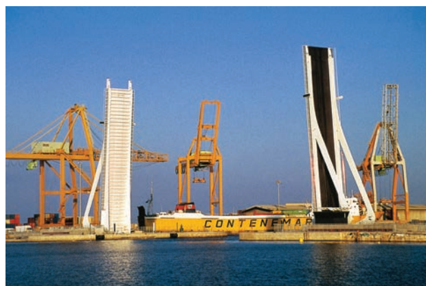
Figura 3. Puente basculante original. Figure 3. Original bascule bridge
