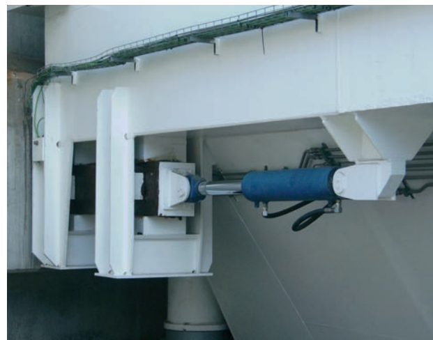
Figura 20. Enclavamiento dorsal. Figure 20. Rear interlocking
