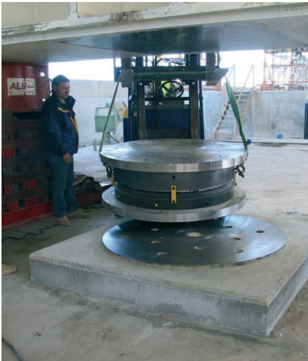
Figura 37. Colocación de la rótula Figure 37. Positioning the turntable gear.
