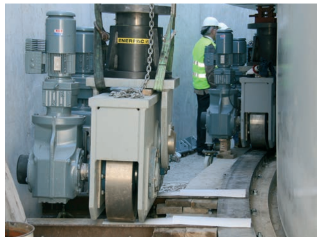
Figura 38. Colocación de carretones Figure 38. Traction wheel installation.
