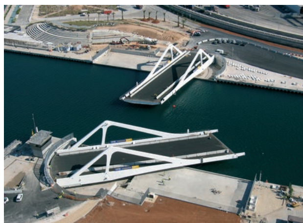
Figura 10. Movimiento de la hoja. Tableros isostáticos. Figure 10. Leaf movement. Statically determinate leaves.
