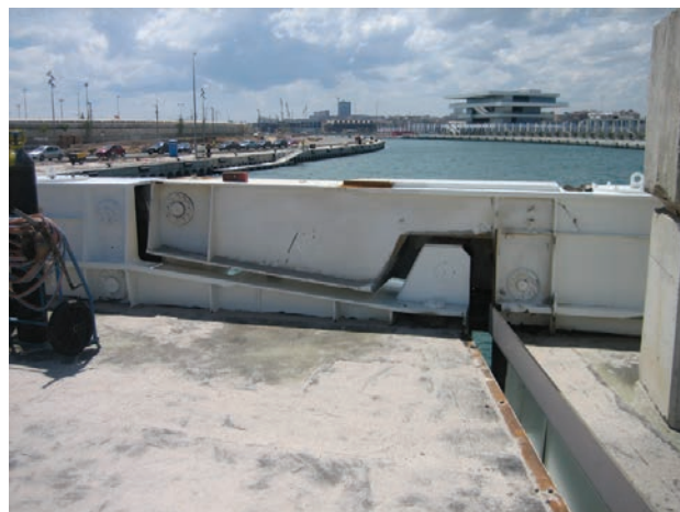
Figura 8. Enclavamiento central. Figure 8. Central interlocking.
