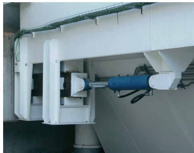
Figura 20. Enclavamiento dorsal. Figure 20. Rear interlocking
