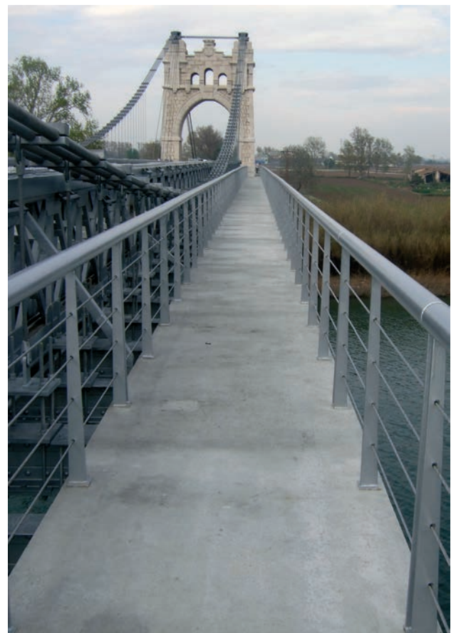
Figura 40. Nueva acera terminada. Figure 40. Finished walkway.
