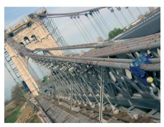
Figura 13. Sistema de cables durante la transferencia inicial de cargas. Figure 13. Cable system during initial load transfer.
