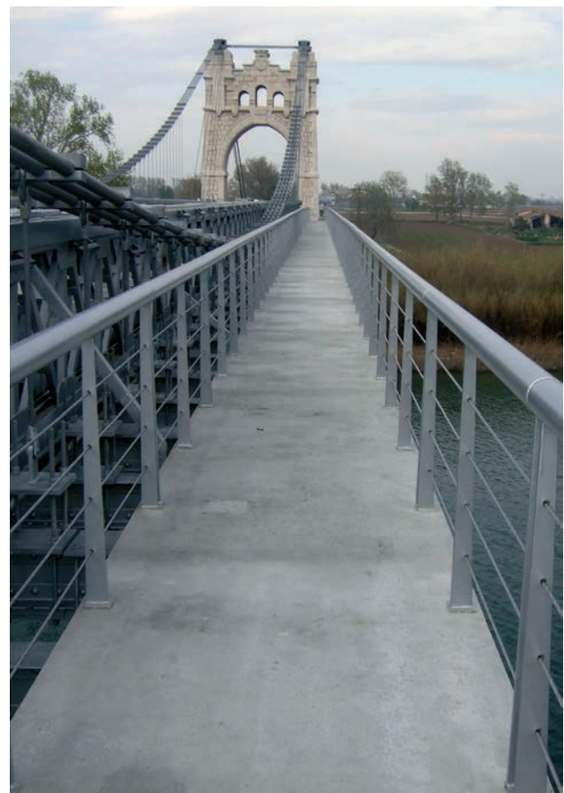
Figura 40. Nueva acera terminada. Figure 40. Finished walkway.
