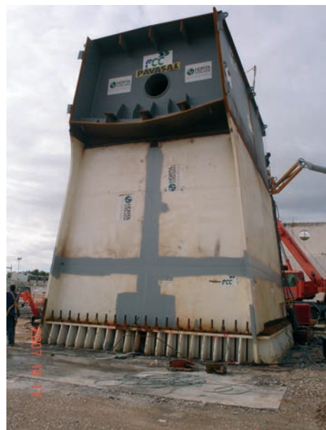
Figura 21. Base. Figure 21. Pier.
