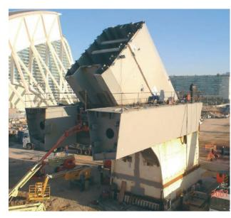
Figure 23. Unión de pilono, tablero y base. Figure 23. Connection of deck, pier and pylon.
