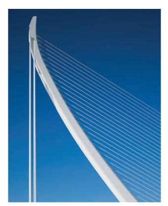
Figura 19. Unión retenida-pilono. Figure 19. Connection between back stays and pylon.
