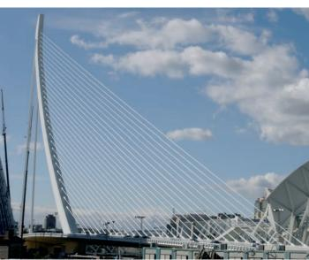
Figura 32. Tirantes y retenida ya tesados. Figure 32. Deck stays and back stays already stressed.
