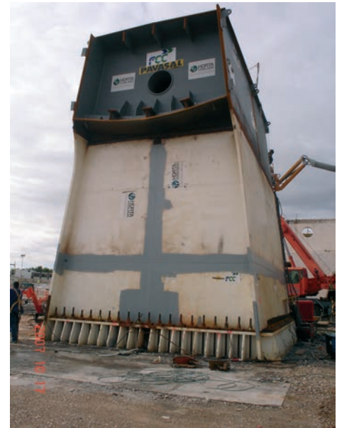
Figura 21. Base. Figure 21. Pier.
