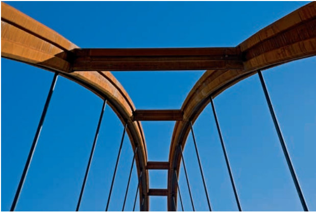
Figura 55. Acabados (I) Figure 55. Finishes (I)
