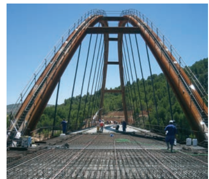
Figura 27. Hormigonado del tablero Figure 27. Laying concrete on the deck
