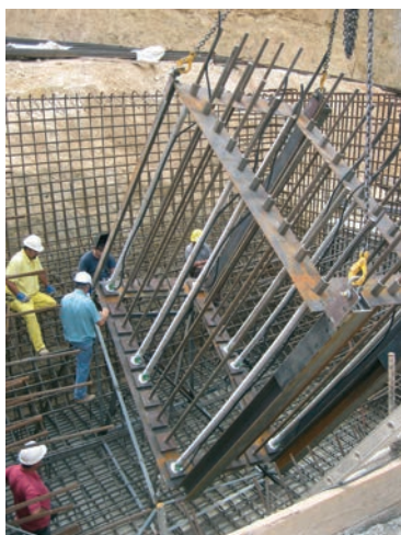
Figura 44. Replanteo de barras Figure 44. Bar stake-out
