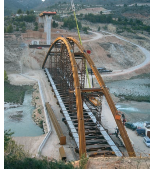
Figura 15. Bowstring (III). Desapeo y péndolas Figure 15. Bowstring (III). De-shoring and hangers
