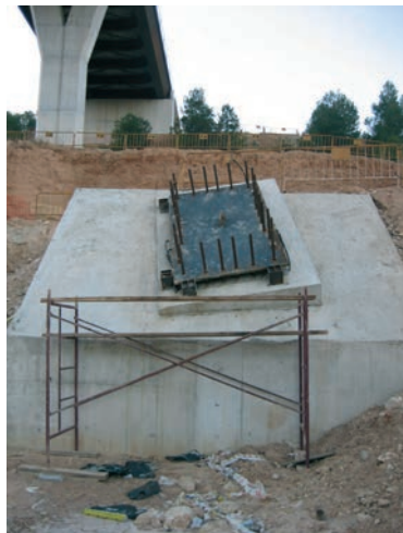
Figura 45. Replanteo placa apoyo Figure 45. Support plate stake-out
