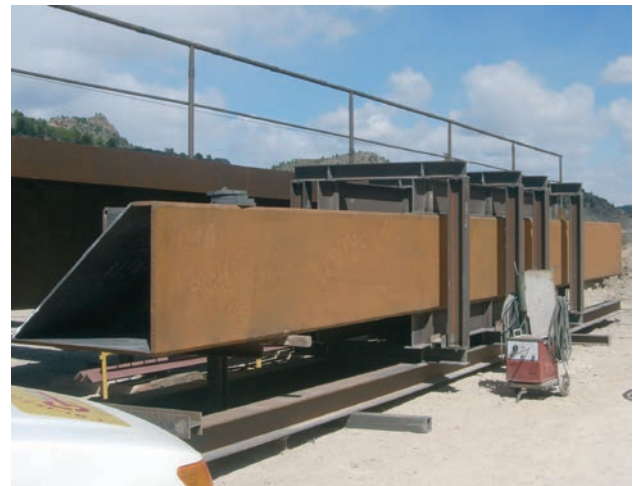
Figura 50. Riostra de voladizo Figure 50. Cantilever brace
