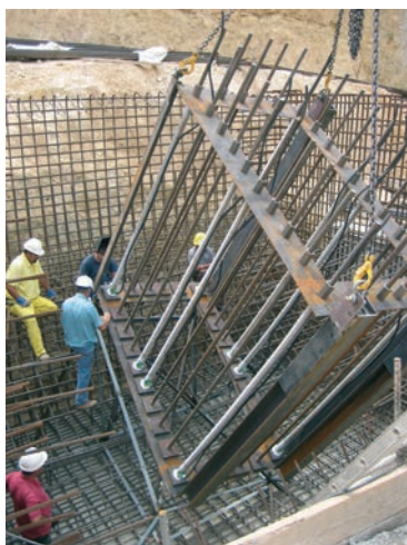
Figura 44. Replanteo de barras Figure 44. Bar stake-out
