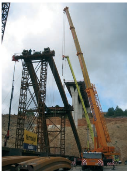
Figura 14. Bowstring (II). Montaje de arco Figure 14. Bowstring (II). Arch assembly
