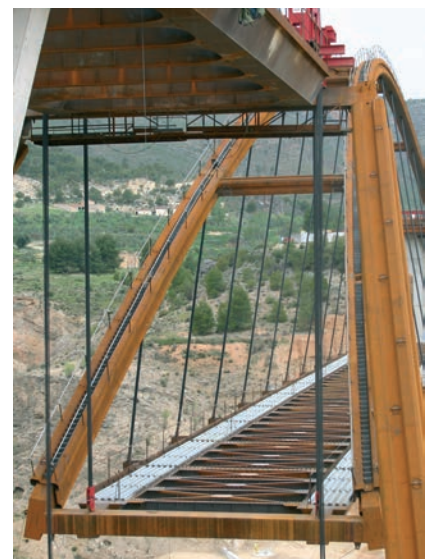
Figure 21. Riostra de bowstring Figure 21. Bowstring brace
