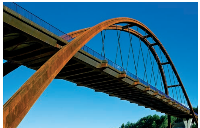
Figura 56. Acabados (II) Figure 56. Finishes (II)
