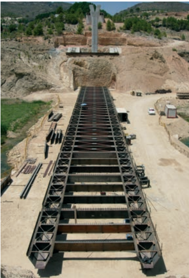
Figura 13. Bowstring (I). Tablero Figure 13. Bowstring (I). Deck
