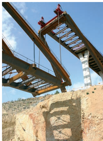
Figura 20. Izado a media carrera Figure 20. Hoisting operation
