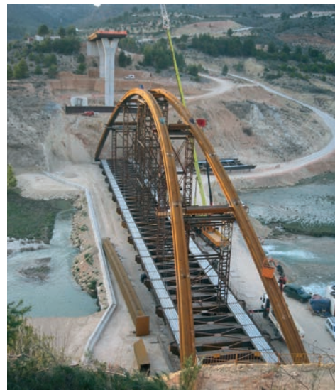
Figura 15. Bowstring (III). Desapeo y péndolas Figure 15. Bowstring (III). De-shoring and hangers
