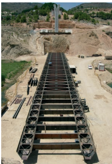
Figura 13. Bowstring (I). Tablero Figure 13. Bowstring (I). Deck
