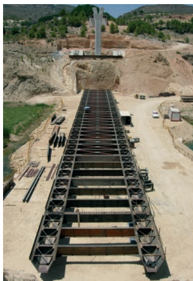
Figura 13. Bowstring (I). Tablero Figure 13. Bowstring (I). Deck
