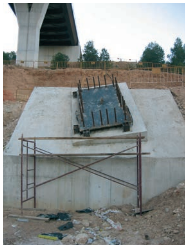
Figura 45. Replanteo placa apoyo Figure 45. Support plate stake-out
