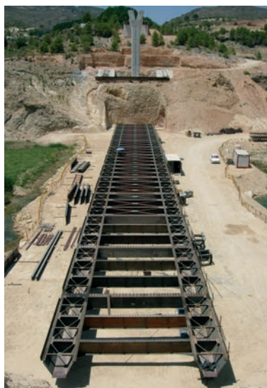
Figura 13. Bowstring (I). Tablero Figure 13. Bowstring (I). Deck
