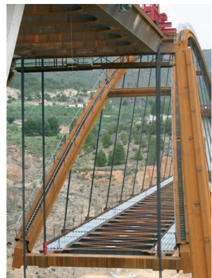
Figure 21. Riostra de bowstring Figure 21. Bowstring brace
