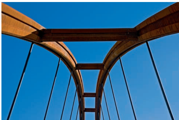
Figura 55. Acabados (I) Figure 55. Finishes (I)
