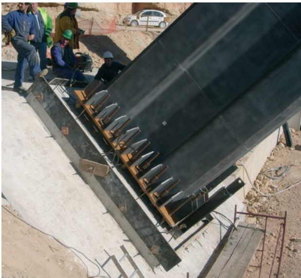
Figura 49. Empotramiento con contratruercas Figure 49. Fixing with grip nuts
