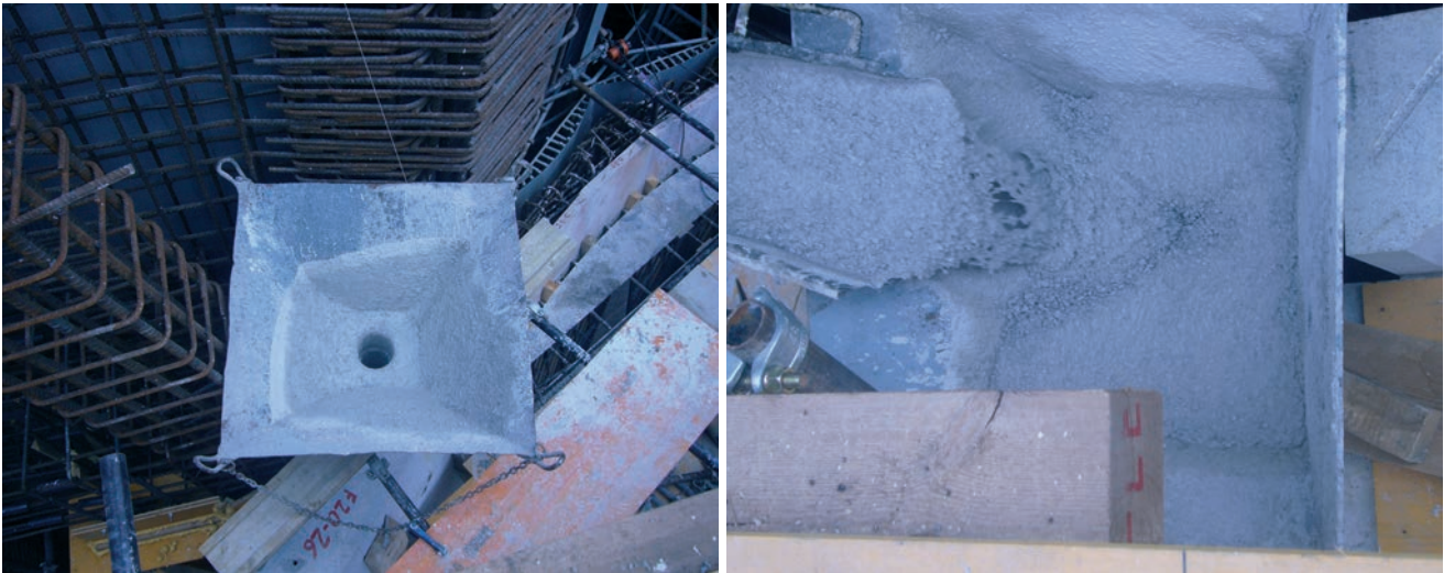
Figura 30. Hormigonado de los muros (a y b). Fuente ATESEF Figure 30. a) and b). Placement of concrete in walls. Source: ATESEF
