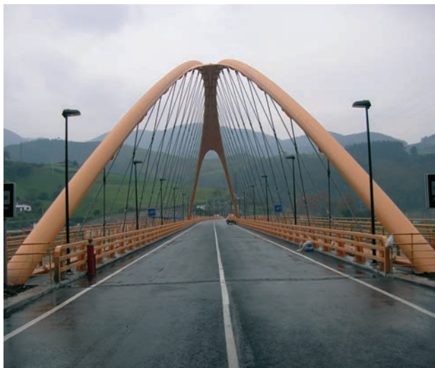
Figura 18. Vista del puente arco desde el estribo 2 (túnel) Figure 18. View of the arch bridge from abutment 2 (tunnel)
