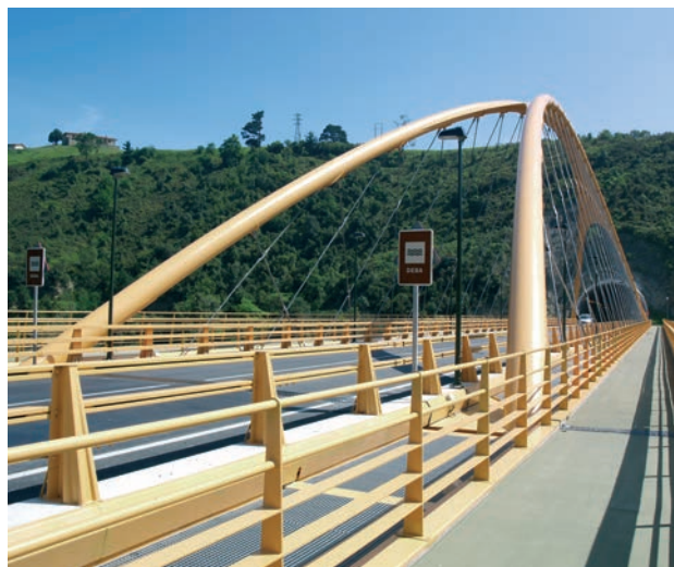
Figura 10. Vista de las aceras voladas laterales Figure 10. View of the lateral sidewalks on cantilever ribs
