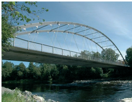
Figura 1. Puente de Steinkjer(1963) Figure 1. Steinkjer Bridge (1963)
