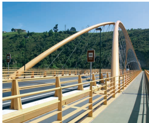
Figura 10. Vista de las aceras voladas laterales Figure 10. View of the lateral sidewalks on cantilever ribs
