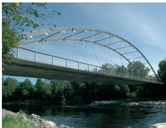
Figura 1. Puente de Steinkjer(1963) Figure 1. Steinkjer Bridge (1963)
