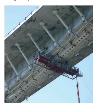
Figura 36. Vista de carro n°2 Figure 36. General view of movable scaffolding n. 2
