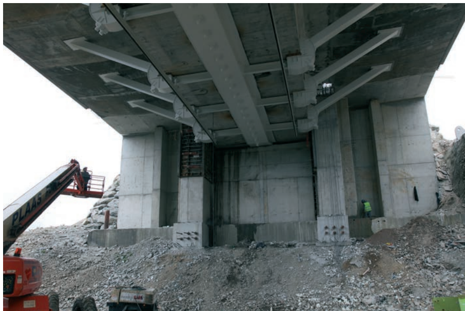
Figura 28. Vista general del estribo una vez reforzado Figure 28. General view of the abutment once it was reinforced
