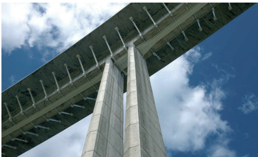
Figura 7. Solución II, refuerzo de cajón existente. Vista inferior del tablero ampliado Figure 7. Solution II, reinforcing of the existing deck. Lower view of the widened deck
