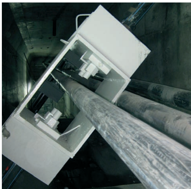
Figura 35. Puente especial para interferencias entre diagonales y pretensado exterior Figure 35. Special steel piece to solve the intersection of the external prestressing tendons with the inclined tensioned bars
