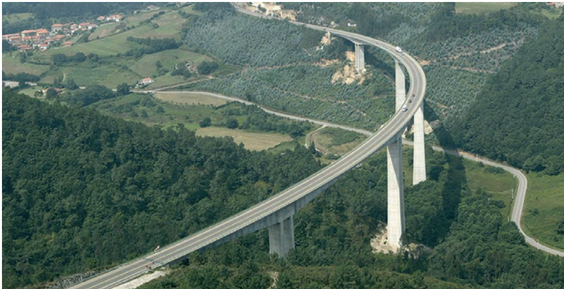
Figura 2. Viaducto original Figure 2. Existing bridge
