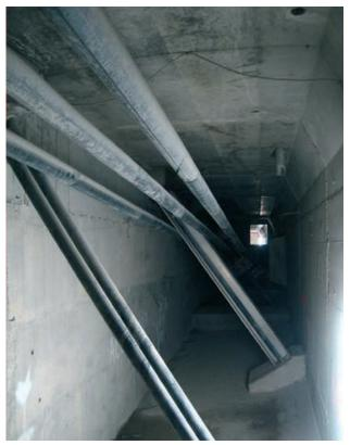
Figura 31. Pretensado longitudinal, diagonales y puntales Figure 31. General view of the external longitudinal prestressing, inlcined tensioned bars and inclined supports
