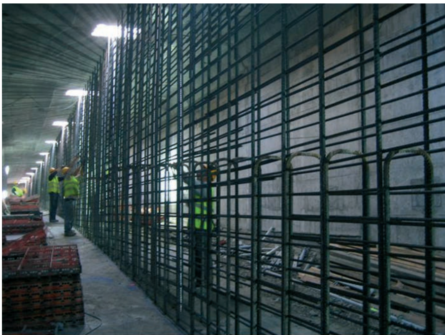
Figura 30. Ferrallado anterior al hormigonado del alma central Figure 30. Installing the reinforcement, before the central web was poured.
