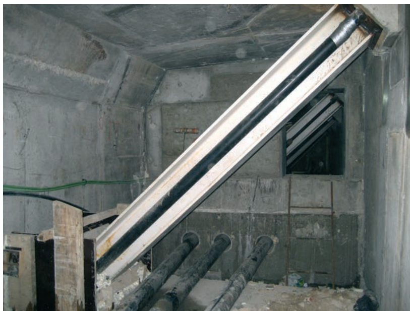
Figura 21. Puntales, diagonales y desviador en centro de vano Figure 21. Inclined internal supports and transverse wall in the centre of the span
