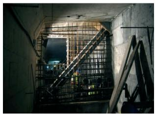
Figura 34. Ferrallado de desviadores Figure 34. Reinforcing of the transvers walls of the deck
