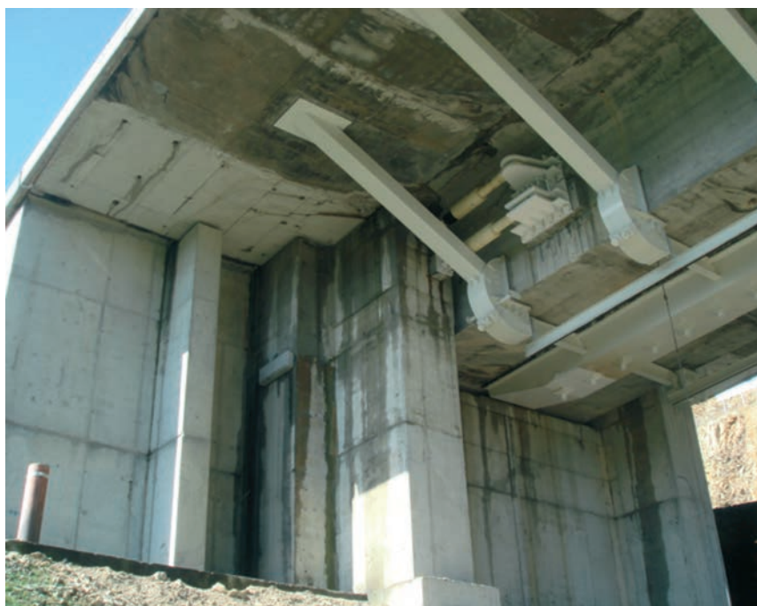
Figura 11. Vista general del estribo y dispositivos transmisores de carga Figure 11. General view of the abutments and of the shock transmission devices
