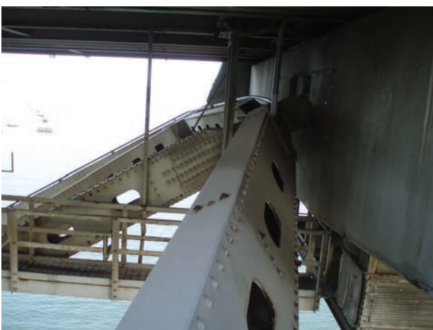
Figura 13. Rótula en plano inferior de celosía Figure 13. Joint on lower truss
