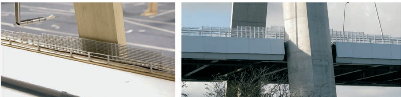
Figura 32. Barandilla alrededor de la torre (modelo y prototipo) Figure 32. Pedestrian guardrail in the neighbourhood of the pylon (model and prototype)
