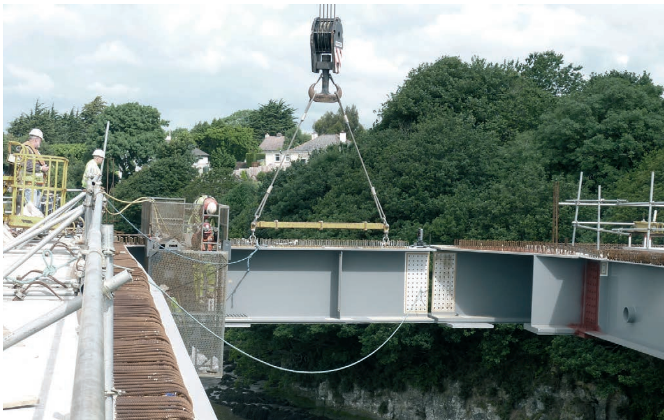
Figura 40. Colocación del tramo de cierre del vano. Figure 40. Installation of the closing segment of the span.
