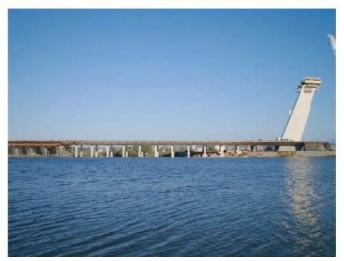
Figura 35. Tablero apoyado sobre pilas provisionales y pilono antes de colocar los cables Figure 35. Deck resting on provisional piers and pylon before cables were strung
