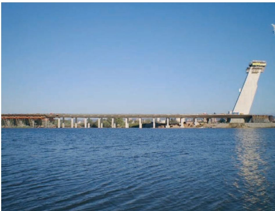
Figura 35. Tablero apoyado sobre pilas provisionales y pilono antes de colocar los cables Figure 35. Deck resting on provisional piers and pylon before cables were strung
