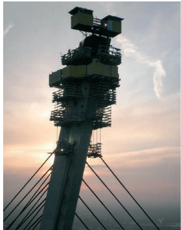
Figura 20. Encofrado autotrepante Figure 20. Self-climbing formwork
