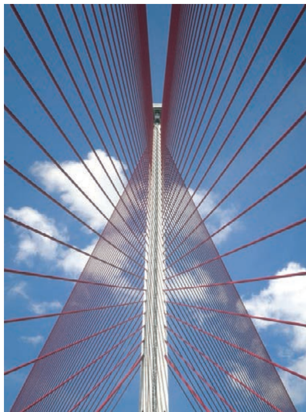
Figura 42. Alzado frontal del pilono con los 152 tirantes Figure 42. Front elevation view of the pylon with its 152 stays
