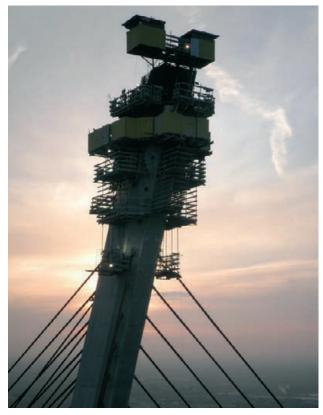
Figura 20. Encofrado autotrepante Figure 20. Self-climbing formwork
