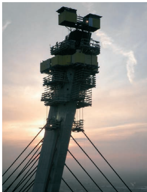
Figura 20. Encofrado autotrepante Figure 20. Self-climbing formwork
