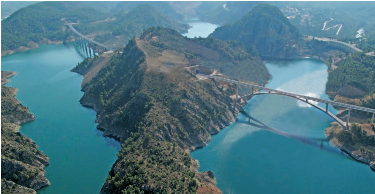
Figura 2. Vista del tramo de ferrocarril de alta velocidad ya construido sobre el embalse de Contreras (se ha eliminado la Autopista) Figure 2. View of the completed high-speed railway line over the Contreras Reservoir. (The Motorway has been removed)
