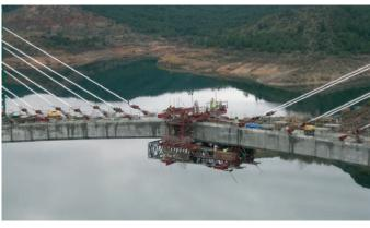
Figure 20. Details of the form traveller and the connection at the key
