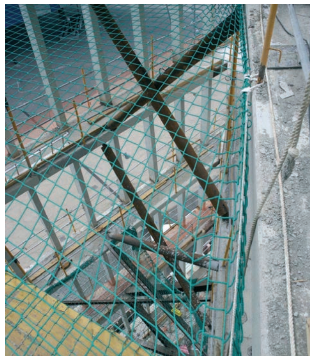
Figura 30. Arriostamiento provisional capa interior fachada en patio Figure 30. Provisional shoring of the inner layer of the facade surrounding the lower patio
