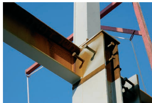
Figura 12. Perfil UPN de borde Figure 12. Edge UPN profile
