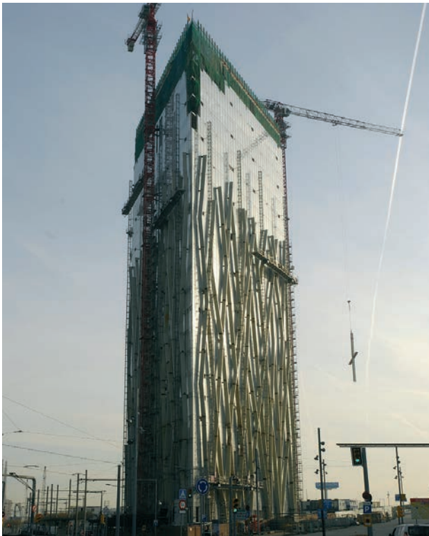
Figura 31. Elevación nudo mediante grúa torre Figure 31. Elevation of a bamboo intersection node by means of the tower crane
