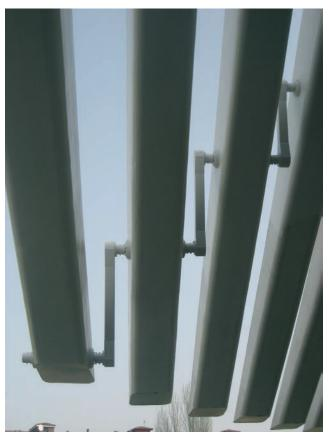
Figura 58. Arriostramientos finalizados Figure 58. Bracing system already finished
