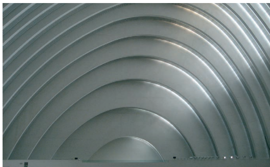
Figura 7. Bóveda superior de la sala mayor del Palacio de Exposiciones y Congresos Figure 7. Top vault of the main auditorium of the Congress and Exhibition Center
