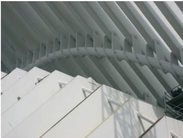
Figura 57. Arco móvil finalizado Figure 57. Moveable arch already finished
