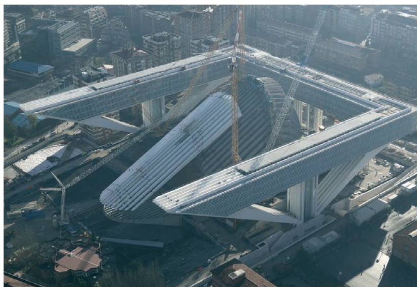
Figura 4. Vista aérea durante las obras del Conjunto de Edificaciones Buenavista Figure 4. Aerial view of the Buenavista Building Complex during the construction works
