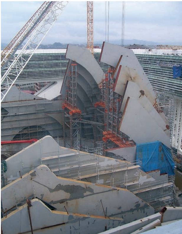
Figura 19. Montaje de las costillas fijas del P.E.C. Figure 19. Mounting stage of the fixed ribs of the Congress and Exhibition Center
