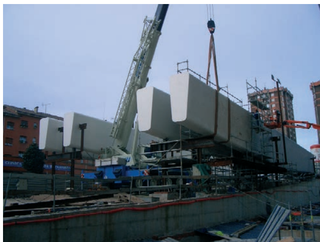
Figura 50. Bancadas de montaje de las costillas móviles Figure 50. Mounting rigs for the moveable ribs
