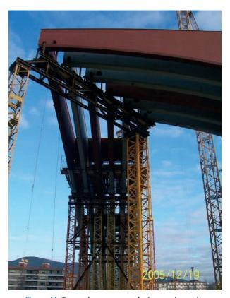
Figura 44. Torres de apeo con celosía superior en las intersecciones Sur-Este y Sur-Oeste Figura 44. Auxiliary supports with upper truss in the South-East and South-West intersections
