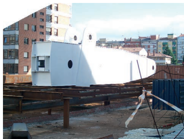
Figura 30. Palanca guiadora antes de ser instalada en el foso Figure 30. Lever arm before its installation in the housing of the cylinders
