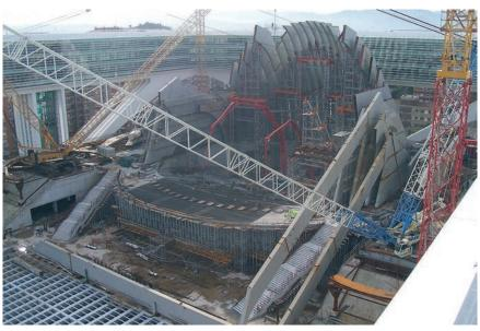
Figura 47. Montaje de las costillas fijas sobre torres de apeo Figure 47. Mounting of the fixed ribs on auxiliary supports
