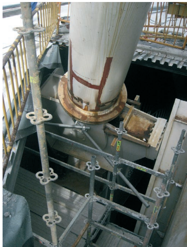
Figura 59. Conexión del extremo inferior del arco móvil a la palanca guiadora Figure 59. Connection of the lower end of the moveable arch to the lever arm
