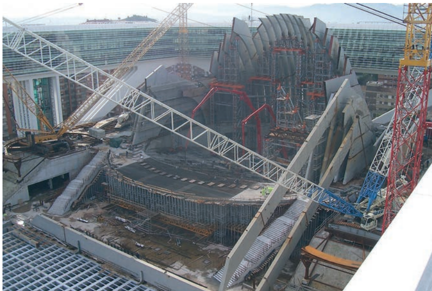
Figura 47. Montaje de las costillas fijas sobre torres de apeo Figure 47. Mounting of the fixed ribs on auxiliary supports
