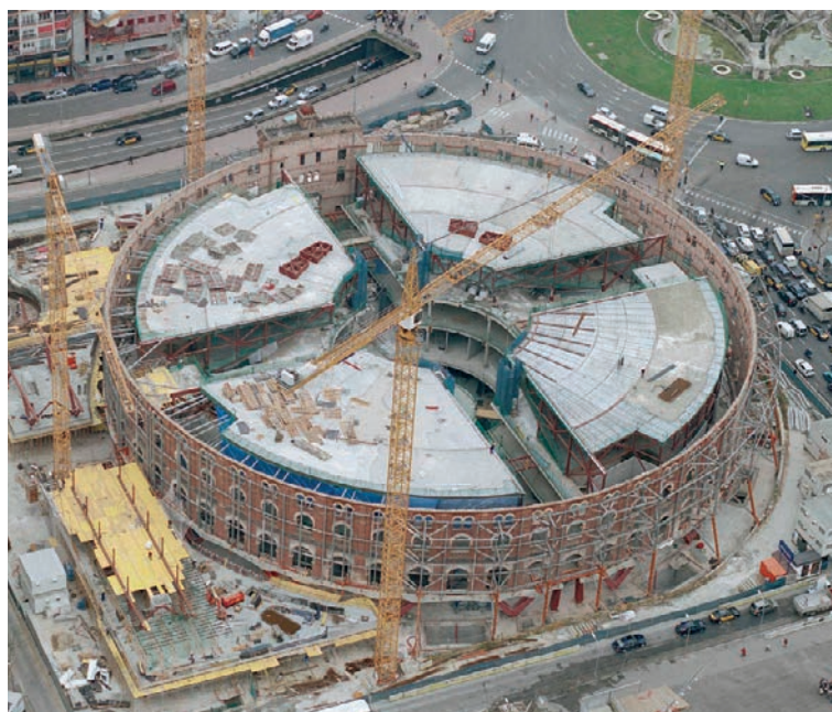
Figura 41. Vista general con el nivel 4 ya hormigonado Figure 41. General view after level-4 concrete was cast
