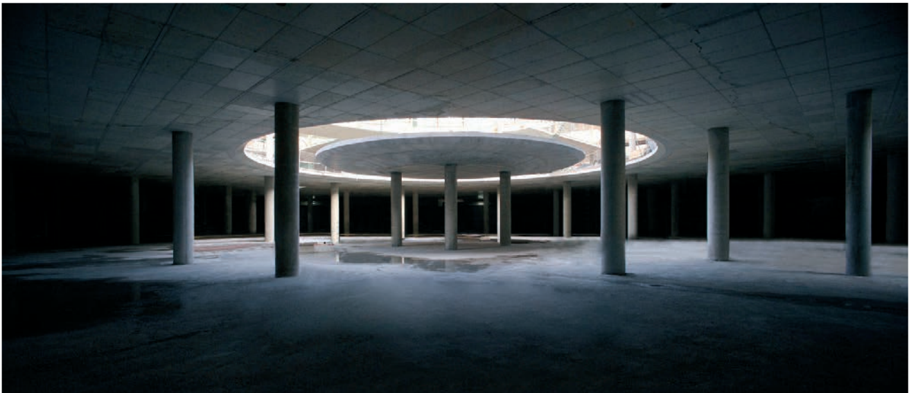
Figura 35. Vista del sótano -1 y de la losa de planta baja con lucernario Figure 35. View of basement level -1 and the ground-floor slab with skylight
