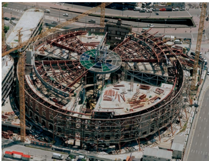
Figura 55. Vista de conjunto con el montaje en diversas fases Figure 55. View of the unit with assembly at various stages
