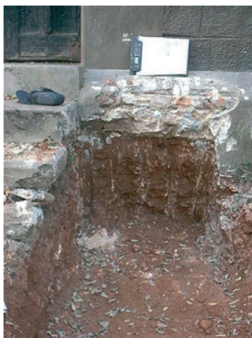
Figura 3. Cata de la cimentación de la fachada Figure 3. Sampling the foundations of the façade
