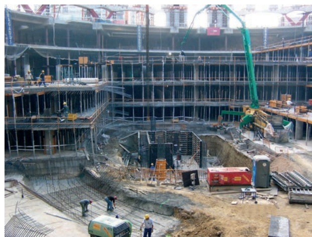
Figuras 36 y 37. Vista general y detallada de la construcción ascendente sectorizada Figures 36 & 37. General and detailed view of upward construction divided into sectors
