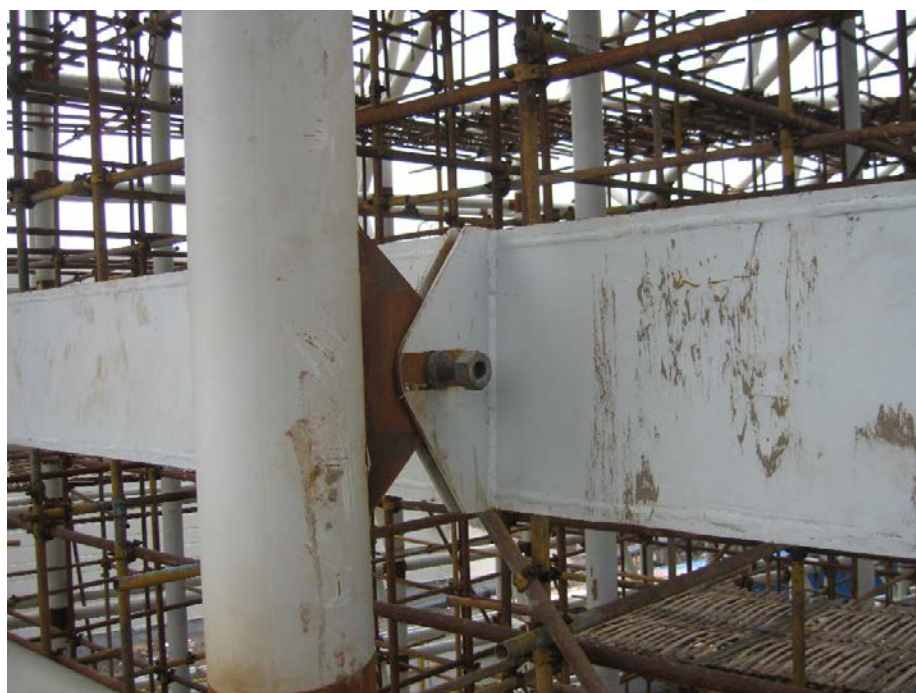
Figura 17. Unión bulonada en construcción, conectando viga de borde con tubo de fachada mediante orejetas Figure 17. Pin-bolt connection under construction, connecting the floor edge beam to the facade tube through ear-plates
