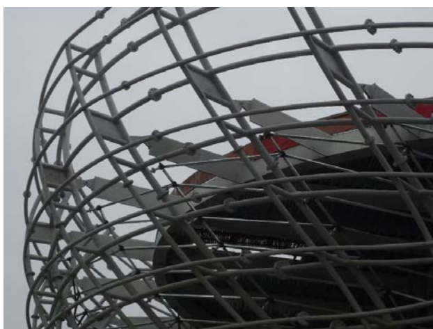
Figura 20. Detalle de la cubierta de la Sala Expositiva 2. Las vigas triangulares se unen por medio de bulones a la fachada, rigidizada por paneles en esa zona Figure 20. Detail of the roof of Exhibition Room 2, where the triangular beams are connected through pin-bolts to the facade, reinforced in this area with plates
