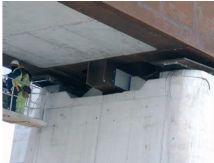
Figura 29. Vista inferior del tope sísmico y aparatos de apoyo en estribo Figure 29. Lower view of the seismic shearkey and bearings at abutments
