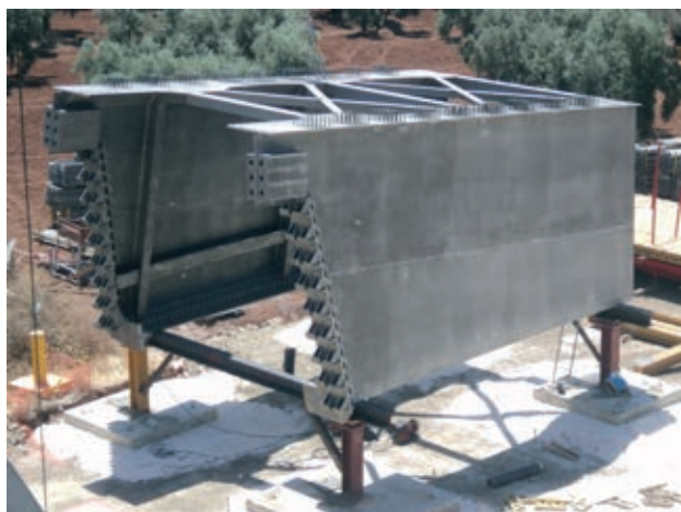
Figura 19. Conexión Pila-Tablero Figure 19. Pier-deck connection
