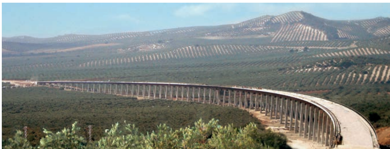
Figura 1. Vista general del Viaducto de Archidona Figure 1. General view of the Viaduct of Archidona
