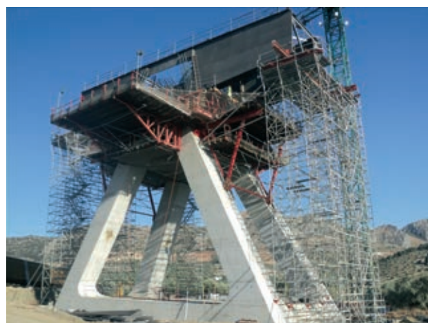
Figura 19. Conexión Pila-Tablero Figure 19. Pier-deck connection
