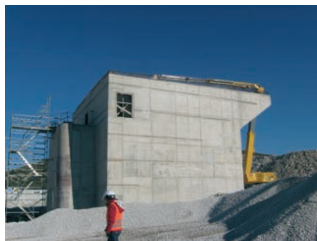
Figura 8. Estribo Figure 8. Abutment
