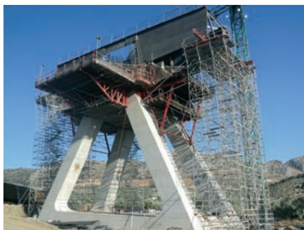
Figura 19. Conexión Pila-Tablero Figure 19. Pier-deck connection
