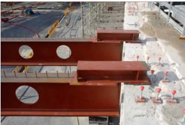
Figure 32. Rabbed skid shoe (during construction).
