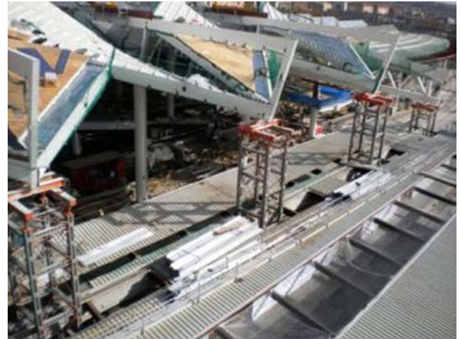
Figure 54. Shoring towers on platform 7.
