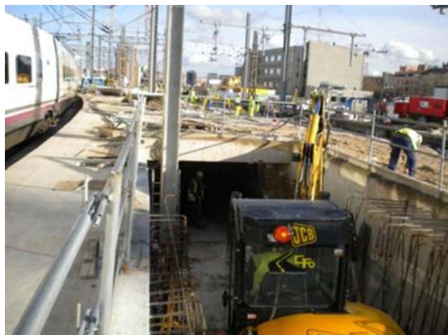
Figure 9. Catering ramps while under construction.
