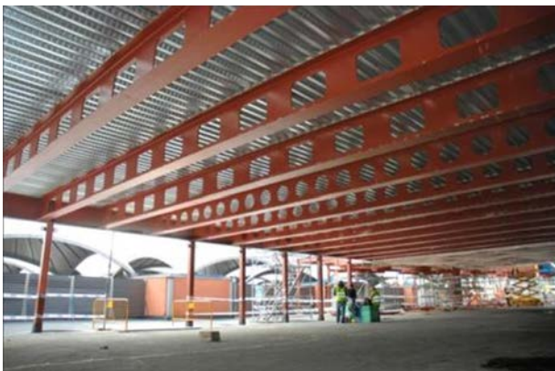
Figure 29. Composite beams with circular openings and "racecourses".
