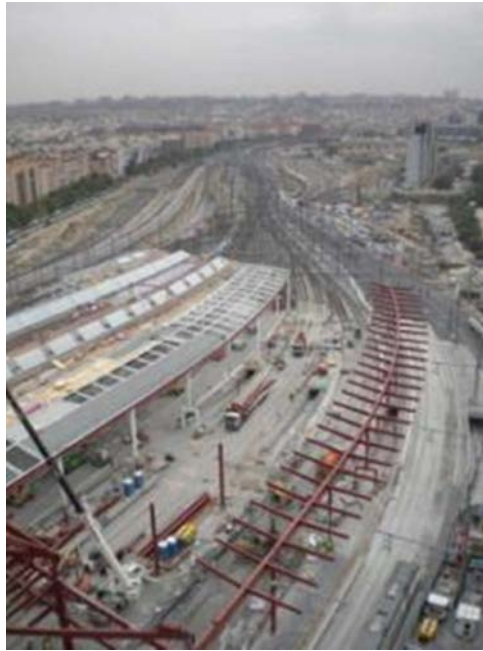
Figure 55. Low-rise canopy construction.
