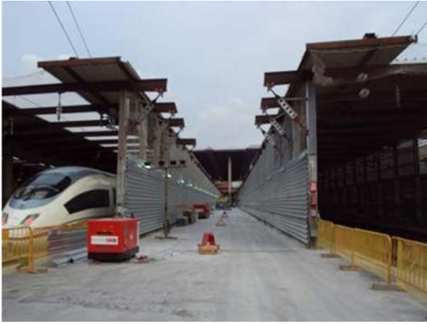
Figure 36. Provisional tunnels to protect tracks.
