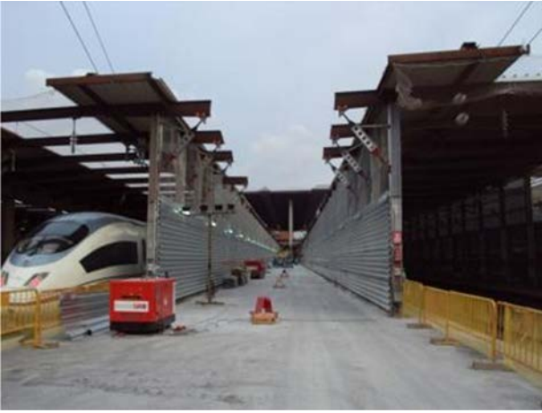
Figure 36. Provisional tunnels to protect tracks.
