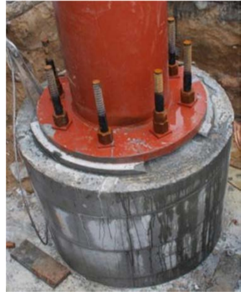
Figure 16. North side low-rise canopy foundations.
