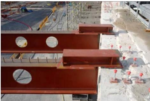
Figure 32. Rabbed skid shoe (during construction).
