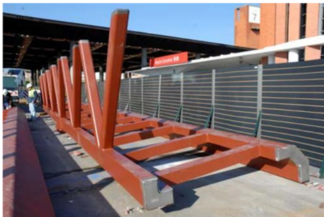
Figure 58. Roof module on the worksite.
