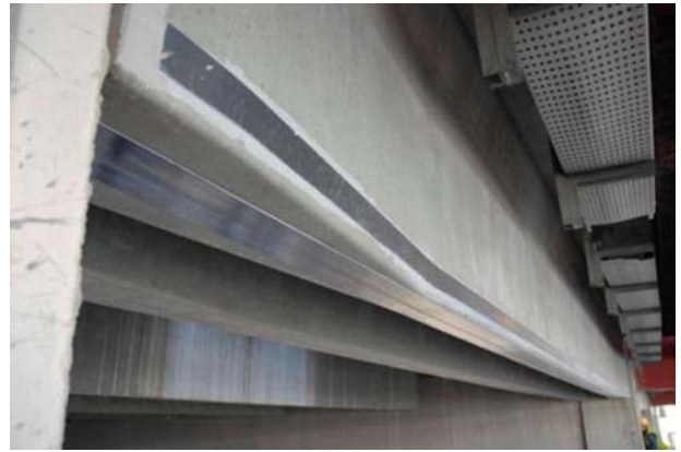
Figure 22. Carbon fibre flexural strengthening for secondary beams.
