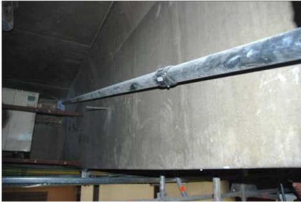
Figure 24. Existing beam strengthened with external post-tensioning.
