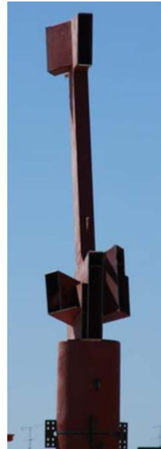
Figure 18. High-rise canopy node during assembly.
