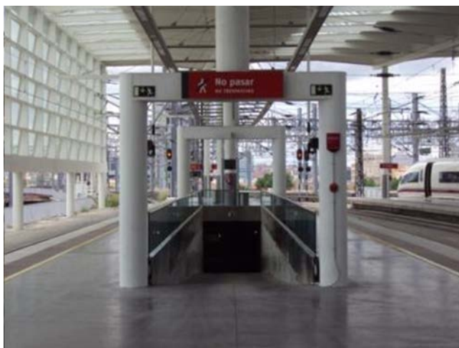
Figure 10. Finished catering ramps.
