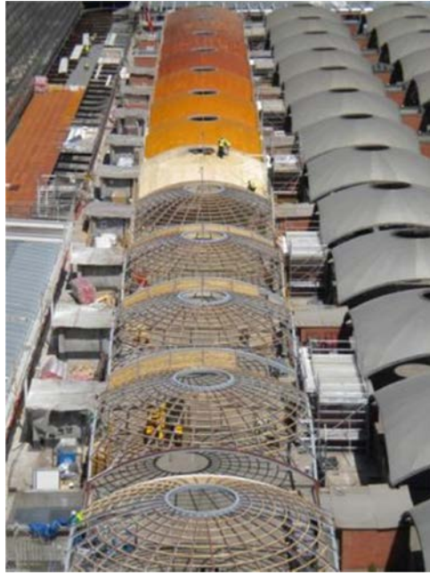
Figure 8. View of domes over the moving walkway during construction.
