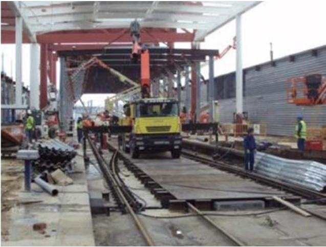
Figure 48. Protection for scissors crossovers.
