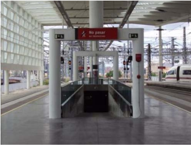
Figure 10. Finished catering ramps.
