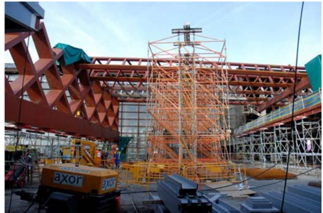
Figure 57. Modular roof construction.
