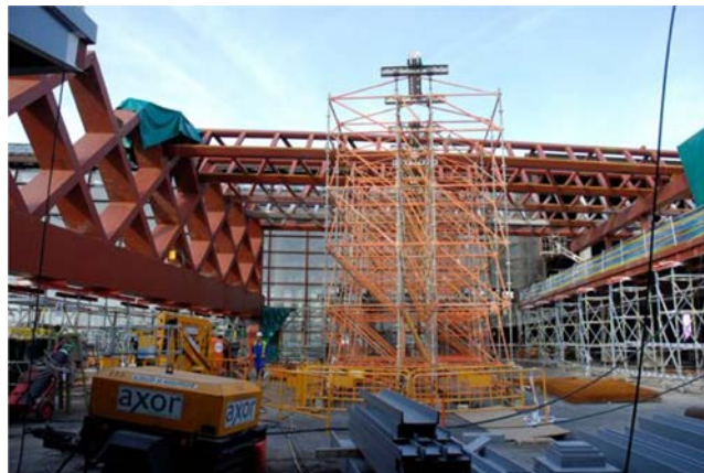
Figure 57. Modular roof construction.
