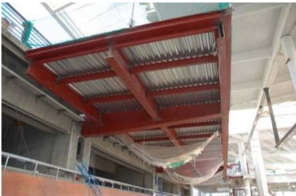
Figure 28. View of cantilevered by-pass from high-speed tracks.
