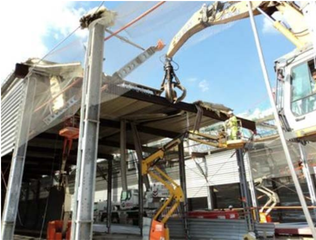
Figure 44. Demolition of provisional tunnels.
