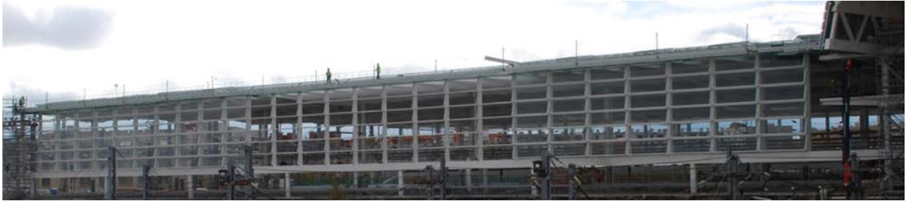
Figure 15. Curtain wall during construction.
