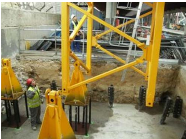
Figure 49. Erecting crane on platform 8.
