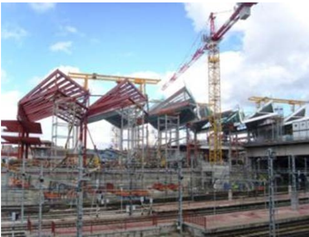
Figure 53. Shoring towers in the local train area.
