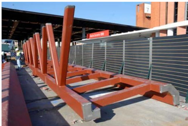
Figure 58. Roof module on the worksite.
