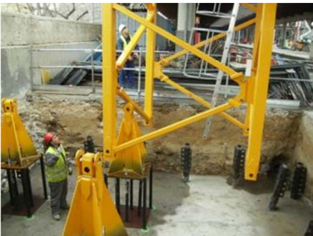
Figure 49. Erecting crane on platform 8.
