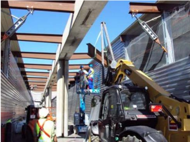
Figure 41. Demolition of canopies between provisional track protection tunnels.
