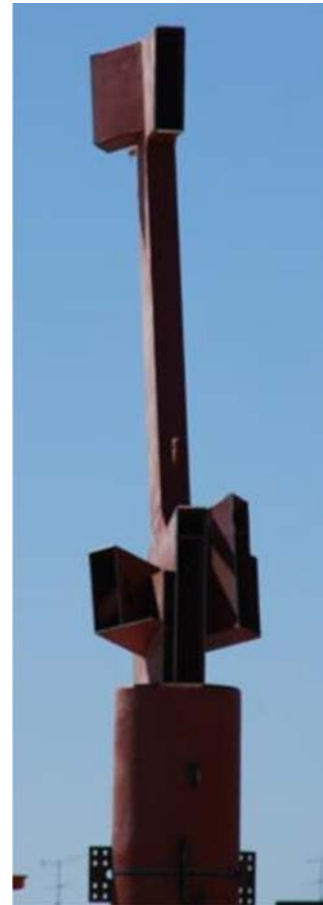
Figure 18. High-rise canopy node during assembly.
