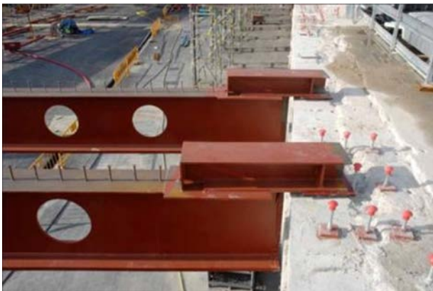
Figure 32. Rabbed skid shoe (during construction).
