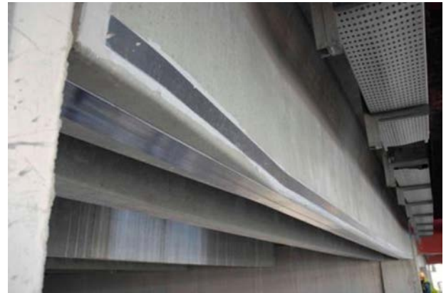
Figure 22. Carbon fibre flexural strengthening for secondary beams.
