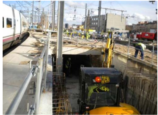
Figure 9. Catering ramps while under construction.
