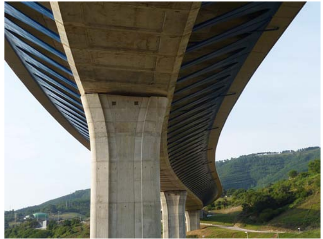
Figure 12. Main viaduct. Lower view.
