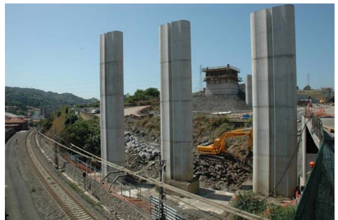
Figure 29. Piers in the transition area.
