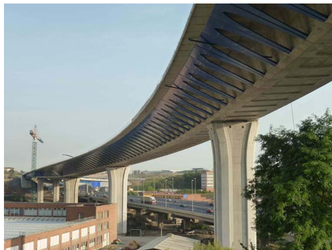
Figure 6. Overall view of the main viaduct.
