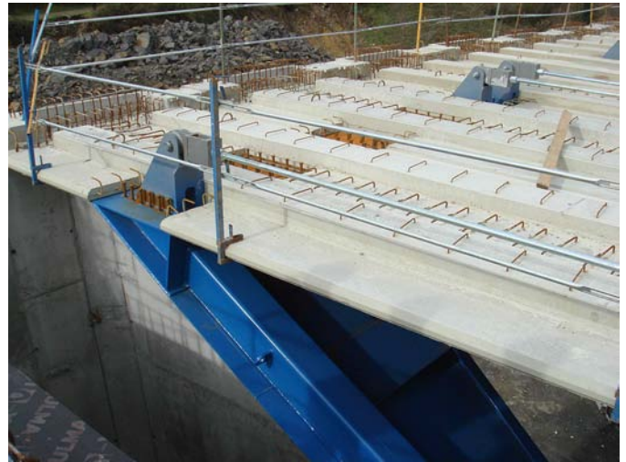
Figure 14. Main viaduct. Placed precast slabs.
