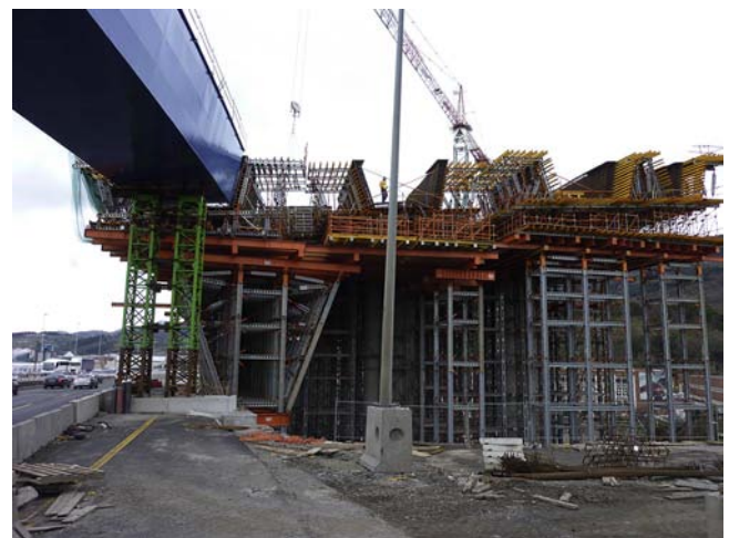
Figures 21 and 22. Views of the falsework in the transition area.
