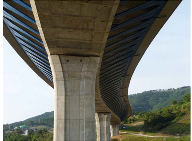
Figure 12. Main viaduct. Lower view.
