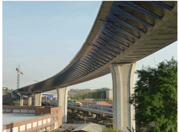
Figure 6. Overall view of the main viaduct.
