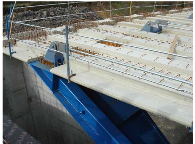
Figure 14. Main viaduct. Placed precast slabs.
