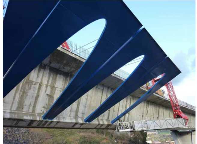
Figure 9. Main viaduct. Lower view of the braced box girders during assembly.
