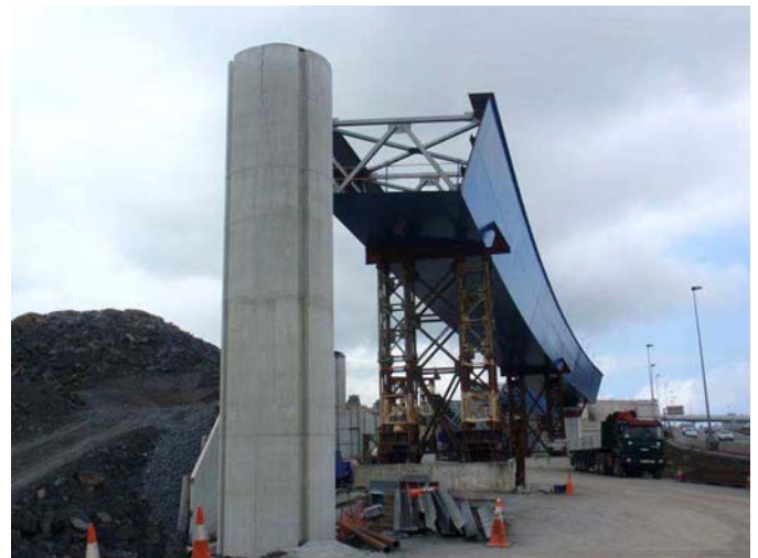
Figure 28. Piers of approach branches.
