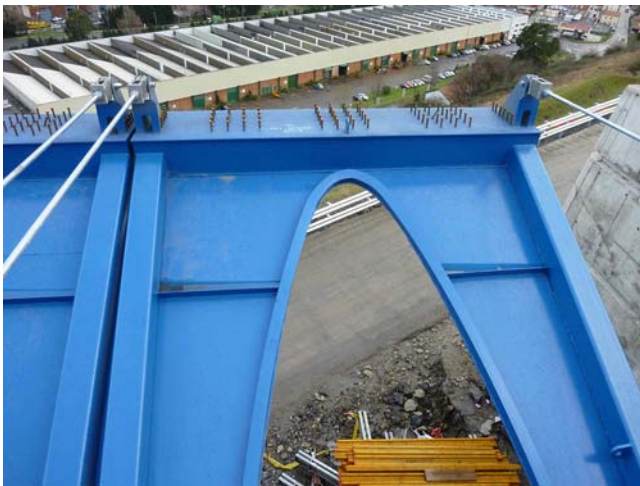
Figures 10 and 11. Main viaduct. Side and front view of the braced box girders.
